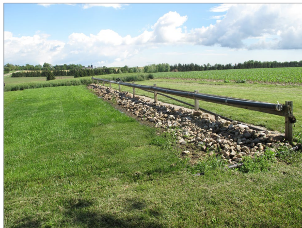
Figure 2. A header pipe with evenly spaced holes (to distribute liquid across the entire width of a vegetated filter strip system) in Middlesex County. The stone base reduces the risk of soil erosion at the start of the vegetated strip.
