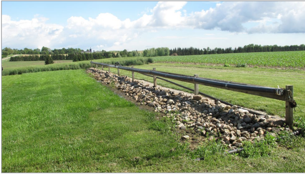
Figure 4. Runoff may be transferred to a vegetated filter strip for treatment.
