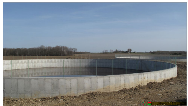
Figure 1. Runoff can be stored in an open-top concrete tank.
