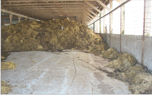
Figure 3. Placing a roof over a permanent solid nutrient storage facility eliminates runoff.
