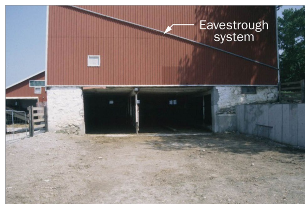
Figure 2. An eavestrough system directs clean water away from the outside yard.
