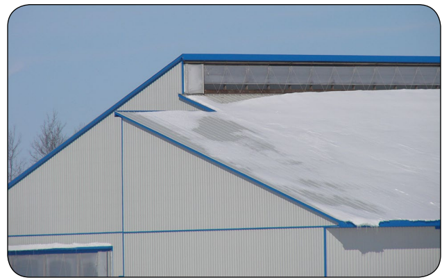
Figure 5. Overshoot roof for ridge exhaust.
