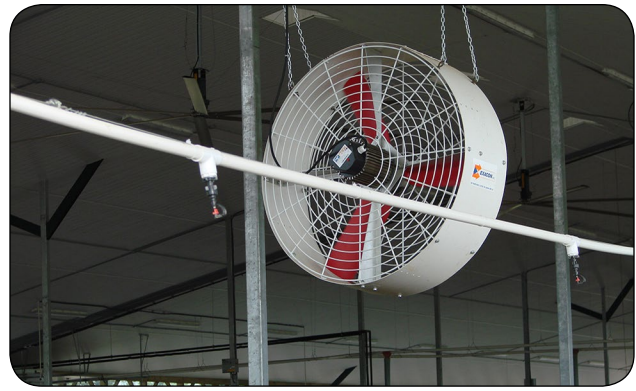
Figure 10. Use sprinklers with fans to wet, then dry the cow for evaporative cooling.
