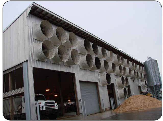
Figure 9. Tunnel ventilation for cooling cows.
