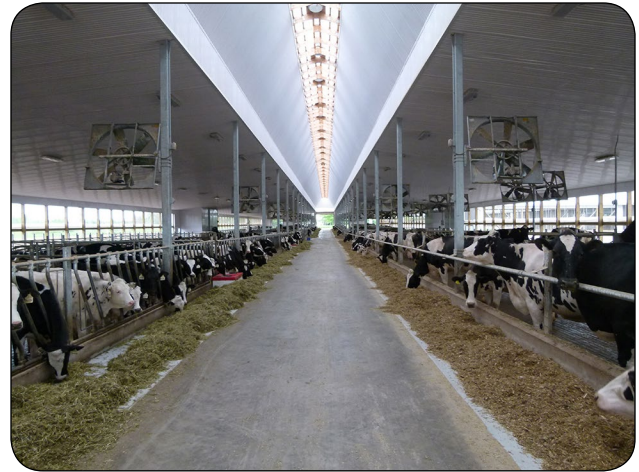
Figure 1. Barn with fully insulated attic.
