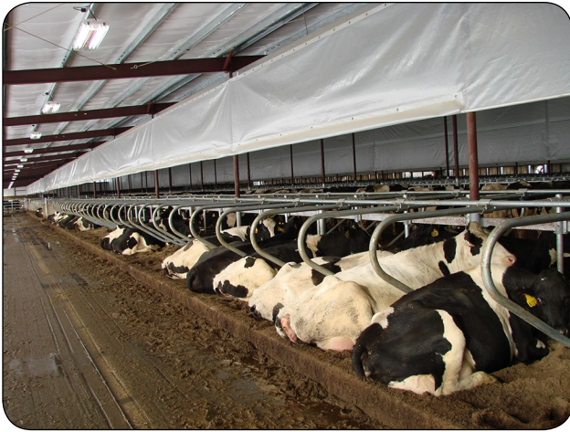
Figure 11. Baffles are used to increase air flow at cow level.
