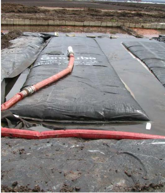
**Figure 8.23. Gros sac filtrant jetable (Geotube®).**
