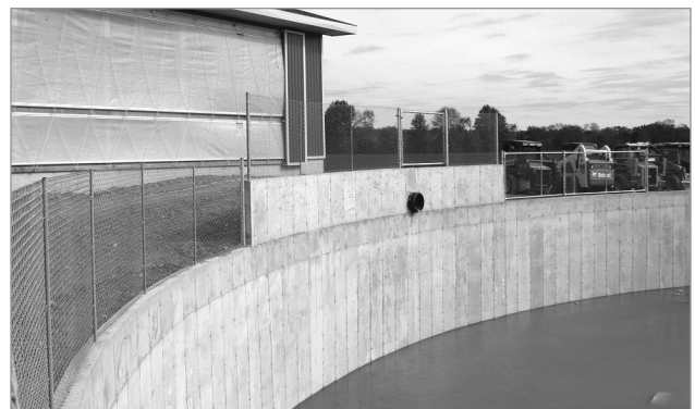
Figure 1. View of a concrete manure storage tank with a 1.5-m (5-ft) high chain link safety fence.
