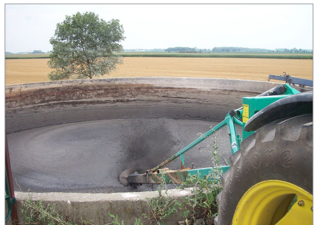
Figure 3. A permanent liquid nutrient storage facility.
