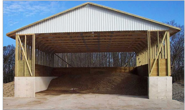
Figure 2. A covered storage reduces or eliminates runoff from solid NASM.
