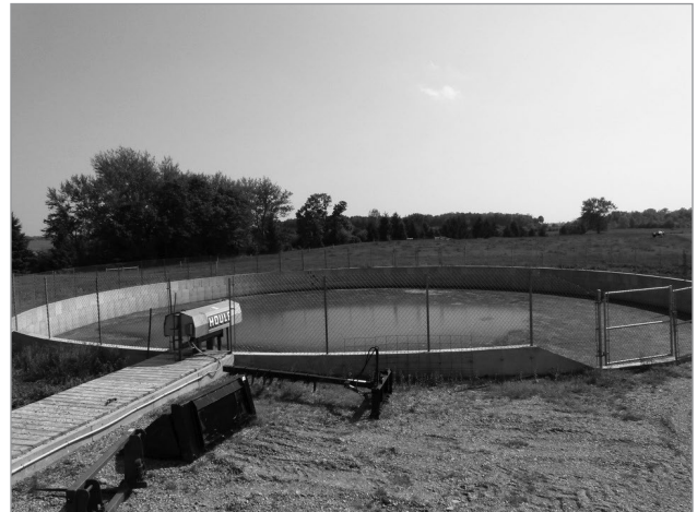
Figure 1. A fenced, reinforced concrete permanent nutrient storage facility built to contain manure and other prescribed material from a livestock operation.
