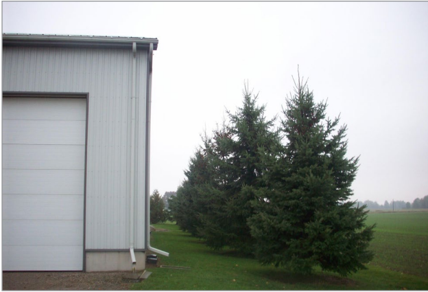
Figure 2. A windswept structure that may not be windswept after the trees grow in height.
