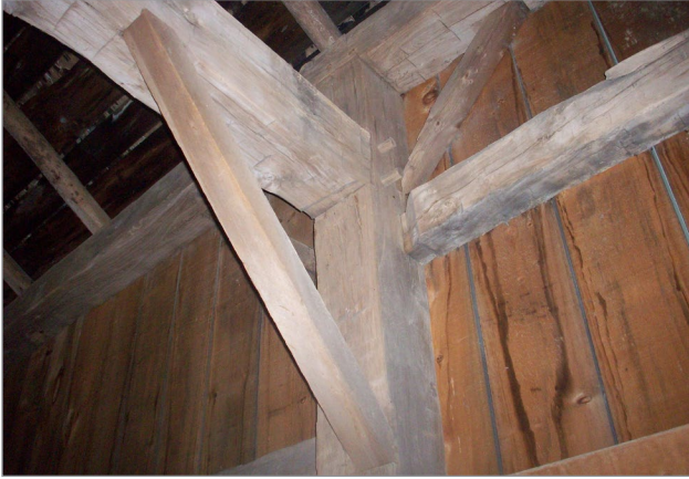
Figure 8. A complex joint in an old bank barn.
