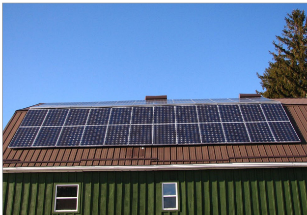
Figure 1. Solar energy is a clean, sustainable approach to producing and using energy in Ontario. Rooftops on rural buildings provide an opportunity for solar photovoltaic (PV) energy generation.
