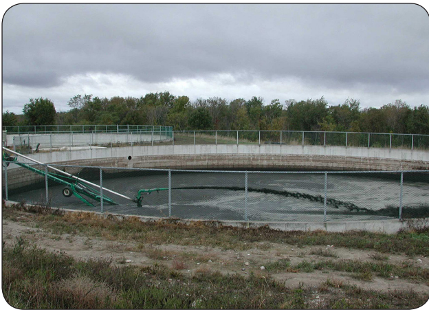
Figure 6. Agitating manure in a concrete storage, 39 m (128 ft) diameter x 5 m (16 ft) deep.
