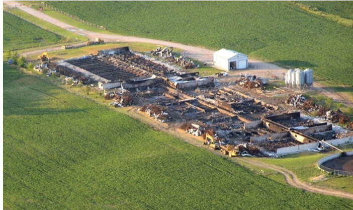
Figure 1.0. This large swine barn was completely destroyed by fire. (Photo credit: P. Stolk, Farm Mutual Reinsurance Plan)
