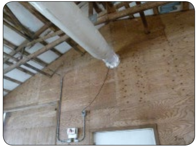
Figure 2. The air tube is sized to match the fan capacity.
