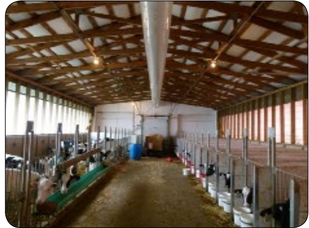
Figure 1. PPAT systems improve calf barn ventilation.
