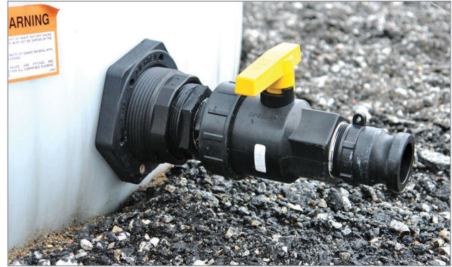
Figure 4. Lightweight ball valve attached to poly tank.
