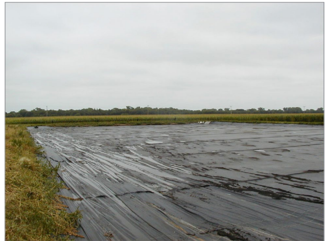
Figure 10. Geotextile floating permeable cover.
