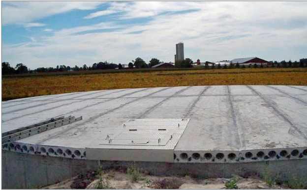
Figure 4. Manure storage with a concrete cover.
