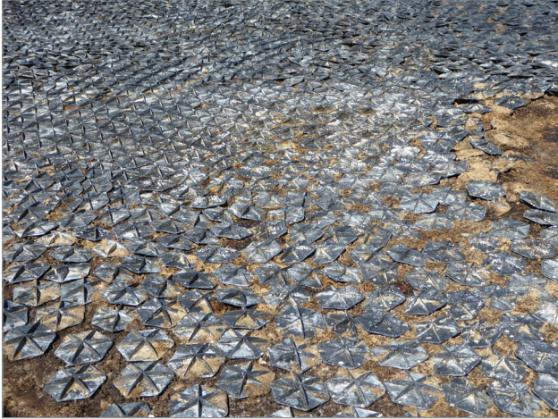
Figure 12. Liquid manure storage permeable cover comprised of plastic hexagon discs.
