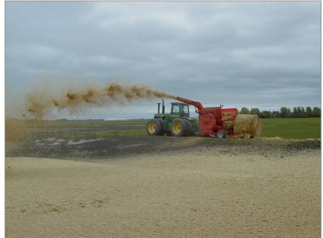
Figure 9. Permeable straw cover.
