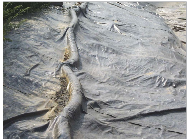
Figure 7. Negative pressure cover being pulled down.
