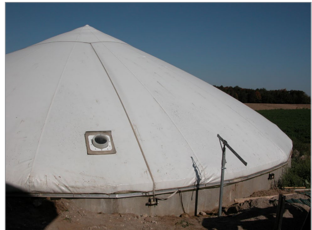
Figure 2. Impermeable positive pressure manure storage cover.
