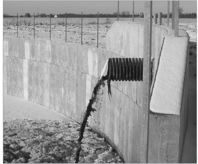
Figure 2. Gravity transfer system discharging over tank wall. Photo credit: Dietrich Engineering Limited.
