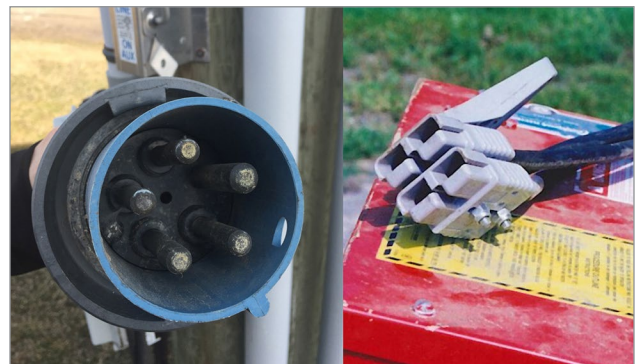
Figure 1. Examples of two types of generator plugs used to connect portable generators on farms. Even if plugs match, DO NOT assume generators can be interchanged between farms.
