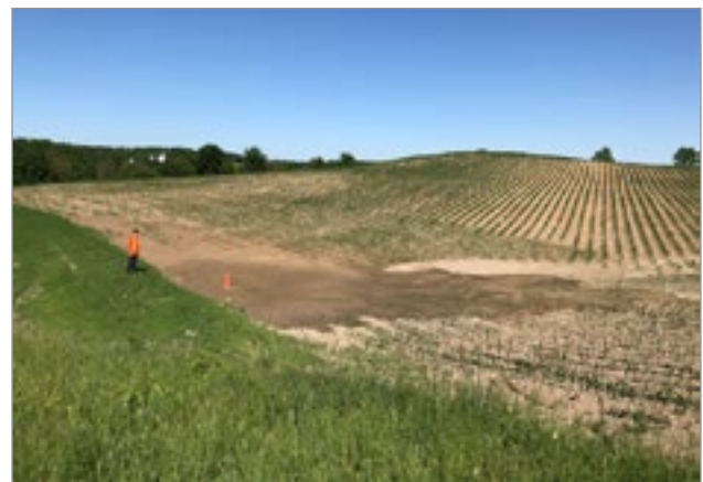
Figure 3. RUSLE2 has the capability to estimate the rate of erosion or deposition at any point along a hill's overland flow path to ultimately estimate the net amount of sediment that is trapped behind this Water and Sediment Control Basin (WASCoB). Source: Grand River Conservation Authority (GRCA), Ontario.
