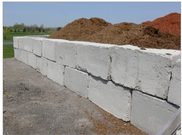
Figure 10. The 0.6 m x 1.2 m x 1.2 m (2 ft x 4 ft x 4 ft) concrete blocks used to build a storage for compost material at this landscaping firm are perfect for building a horse manure storage.
