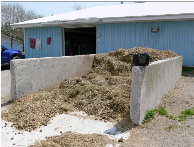
Figure 9. This 3 m x 6 m x 1 m high (10 ft x 20 ft x 3.25 ft) horse manure storage has reinforced concrete walls, making it easy to push against with a loader.
