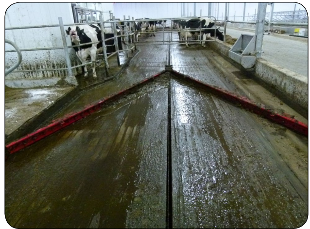
Figure 4. Alley tube scraper pulls manure to a centre slot.
