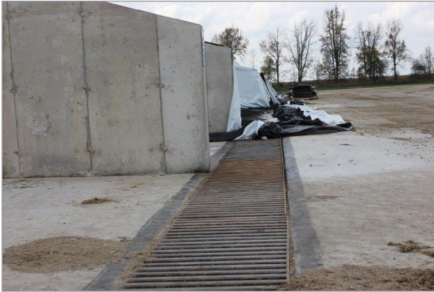
Figure 6. Collection trench in front of an empty bunker.
