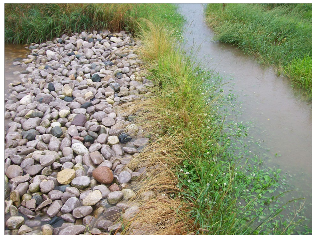
Figure 5. Emergency spillway between holding pond and vegetated flow path.
