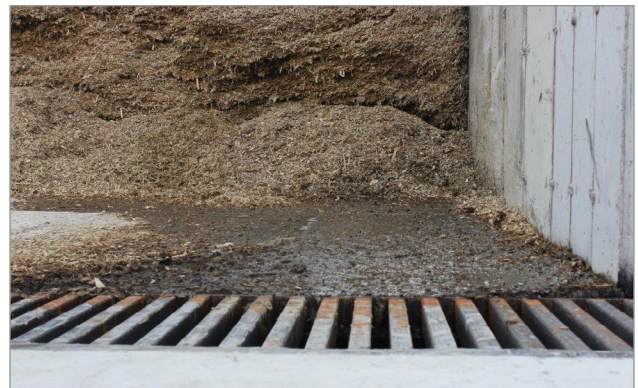
Figure 1. Silage effluent seeping into a collection trench.
