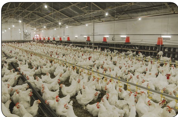
Figure 1. LEDs in use in a poultry facility. Source: Energywisegroup.com.au .
