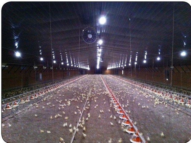
Figure 5. A poultry barn with 12W LED lighting spaced at 3.6 m (12 ft). Source: www.poultryventilation.com .
