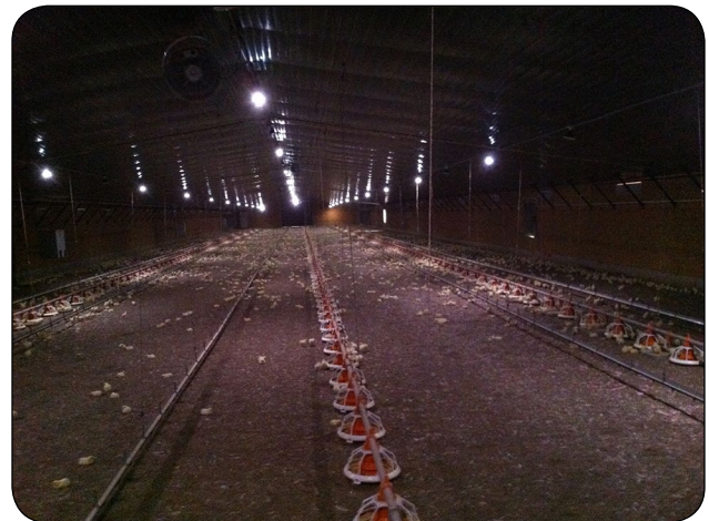
Figure 6. A poultry barn with 12W LED lighting spaced at 7.3 m (24 ft). Source: www.poultryventilation.com .
