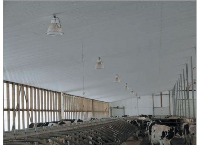
Figure 2. Uniform light levels should be maintained in areas where the cows are active.
