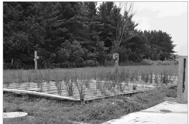
Figure 6. This three-celled engineered wetland treats milking centre washwater from a dairy goat operation as well as runoff from the adjacent 280-m 2 solid manure storage facility.
