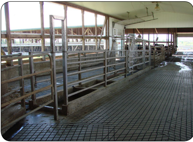
Figure 3. Diamond grooving for improving traction.
