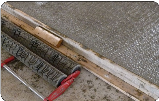
Figure 1. Jitterbug for producing textured surface.
