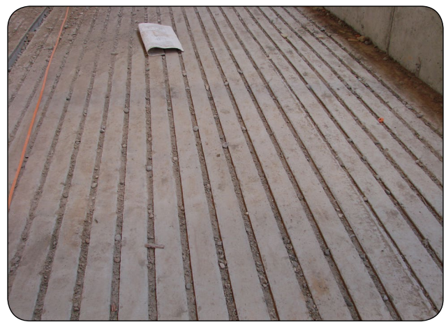
Figure 2. Longitudinal grooves for improving traction.
