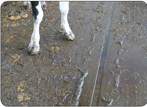
Figure 4. Surface milling improves traction.
