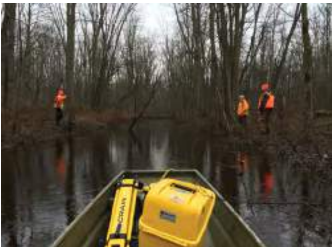
Figure A3-2. Inspection et levé du drain. Source : Dietrich Engineering Ltd., Kitchener, Ontario
