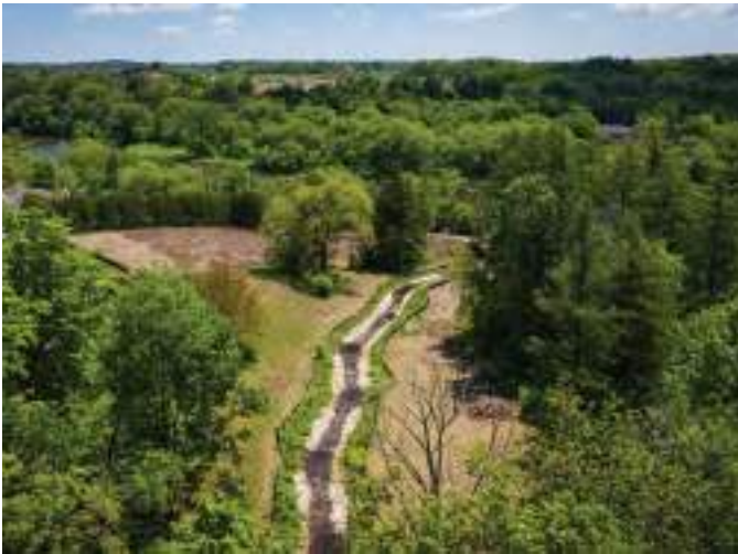
Figure B4-27. Native vegetated sod mats – installed along a drain.
