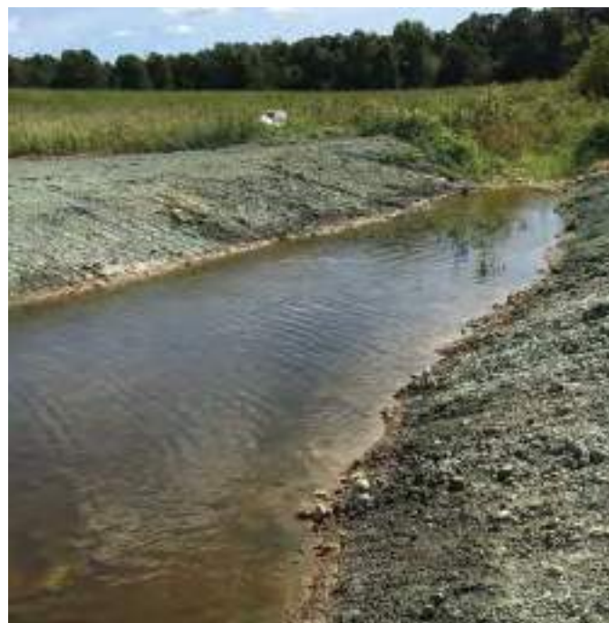
Figure A3-16. Hydro-seeding on both banks of a drain.
