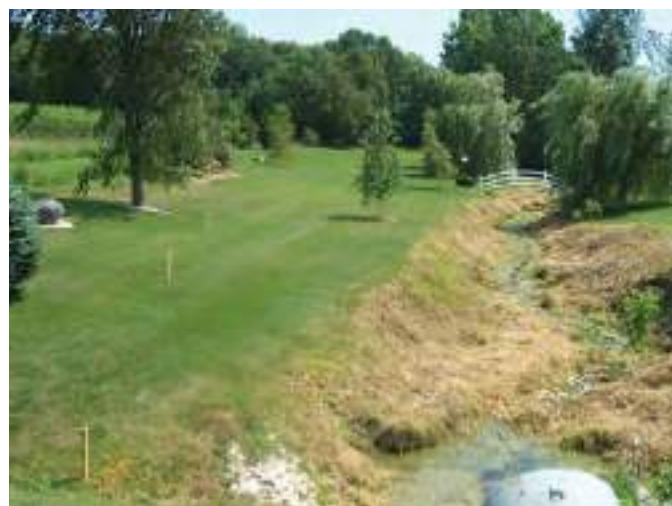
Figure B5-2. Steenstra Drain – Condition of the Drain in 2005.
