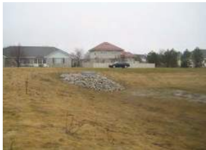
Figure B4-40. A dry pond. Source: Dietrich Engineering Ltd., Kitchener, Ontario
