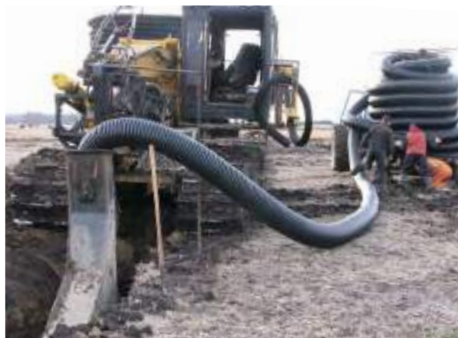
Figure A6-3. Installation of tile drainage.
