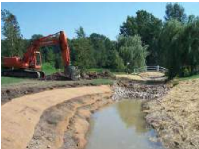
Figure B5-8. Steenstra Drain – Construction. Source: Municipality of Central Huron, Ontario
