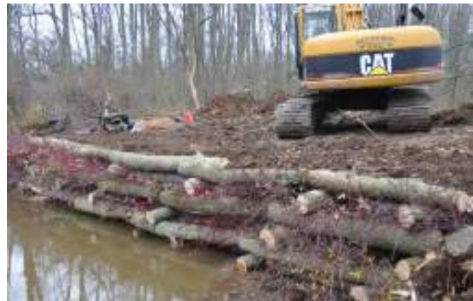
Figure B4-19. Construction of a live cribwall.
