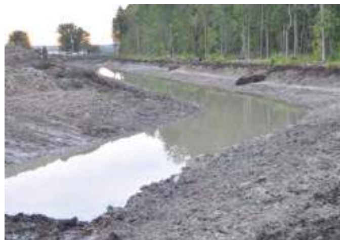
Figure B4-17. A dewatered channel with a littoral shelf on the right side of the channel. Source: K. Smart & Associates Ltd., Kitchener, Ontario
