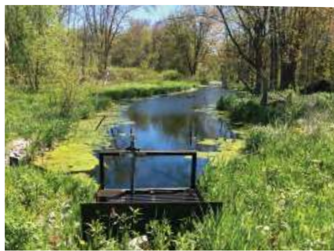
Figure B5-17. Dry Creek – after restoration, the creek now retains water in the restored wetland.
