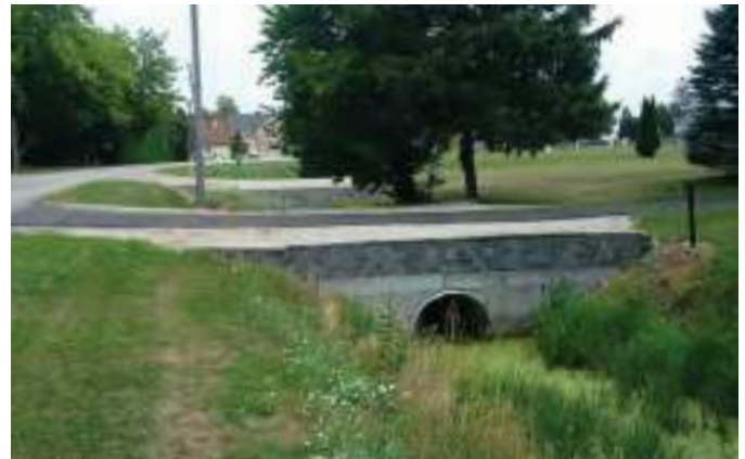
Figure A2-2. Crossing with decorative end wall. Source: Municipality of Chatham-Kent, Ontario
