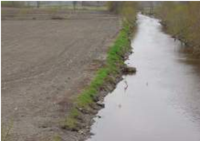
Figure A4-5. Damage to a municipal drain by the removal of a buffer that was incorporated into the drain by the engineer’s report and bylaw.
