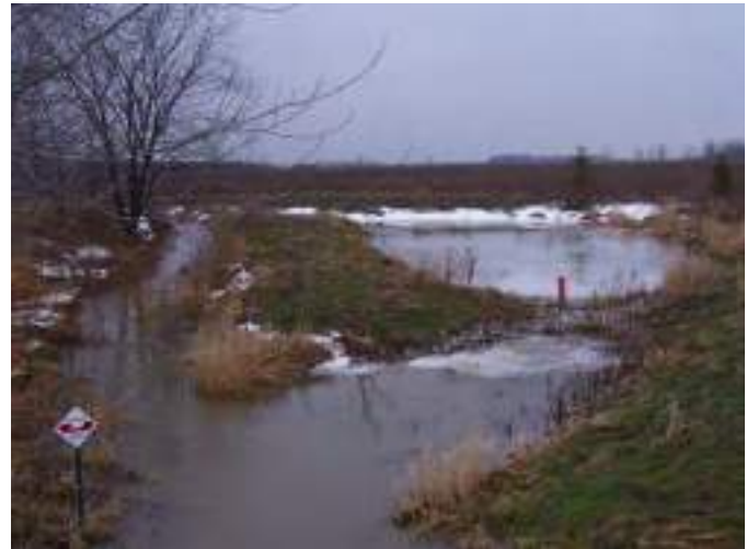
Figure B5-6. Steenstra Drain – Constructed sediment trap. Source: Municipality of Central Huron, Ontario
