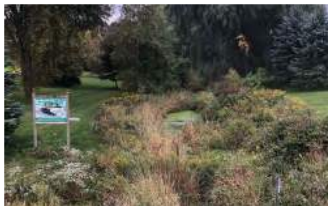
Figure B5-3. Steenstra Drain – Bioengineered channel bank for protection and habitat (2020).
