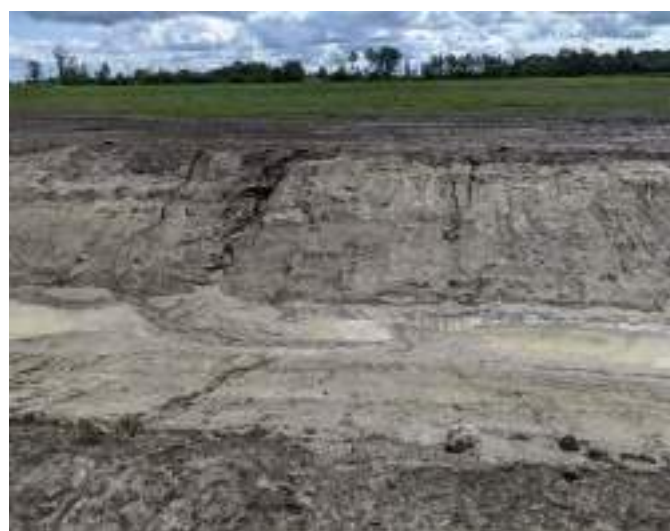
Figure B4-6. Soil erosion resulting from not maintaining a vegetated cover (barren soil). Source: City of Kawartha Lakes, Ontario.
