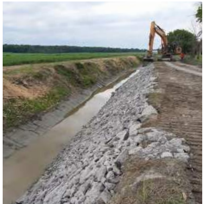
Figure B4-31. Riprap armouring of a drain.
