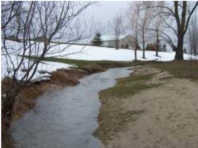
Figure B5-4. Steenstra Drain – Sediment issues caused by highly erodible soils. Source: Municipality of Central Huron, Ontario
