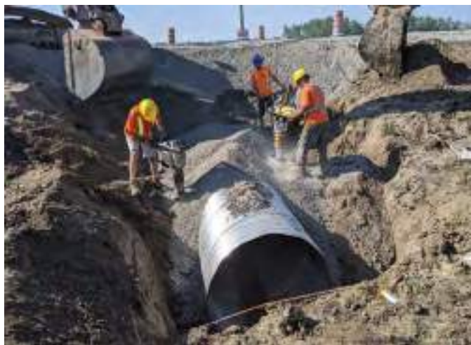
Figure A3-7. Backfilling around a new culvert.
