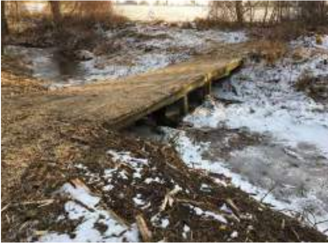
Figure A4-3. A low bridge over a drain that may cause an obstruction.
