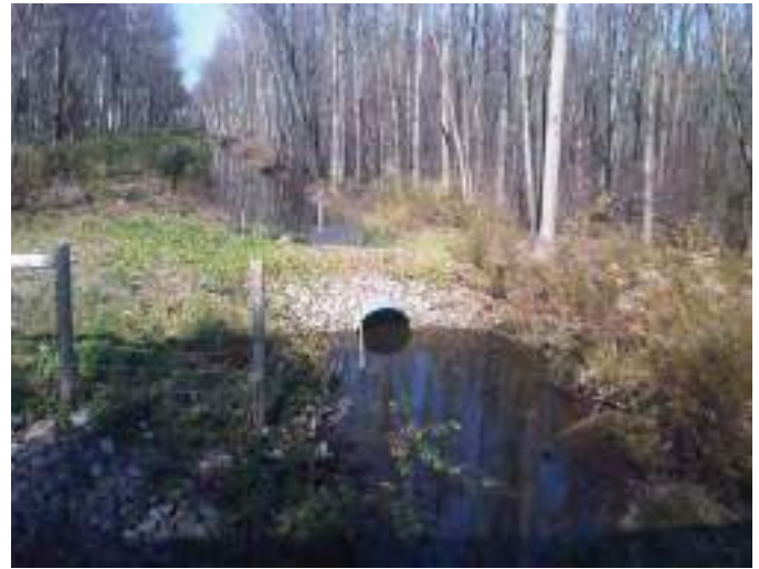
Figure B4-12. A wetland enhancement project.
