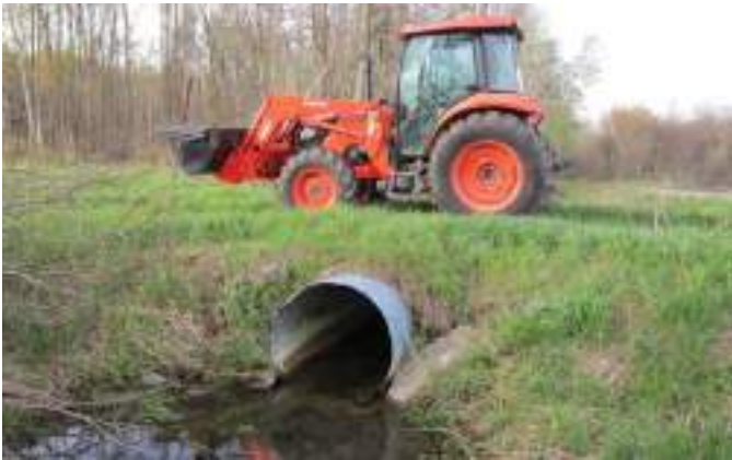
Figure A3-26. Farm crossing over a drain to allow access to a portion of the property due to the presence of the drain.
