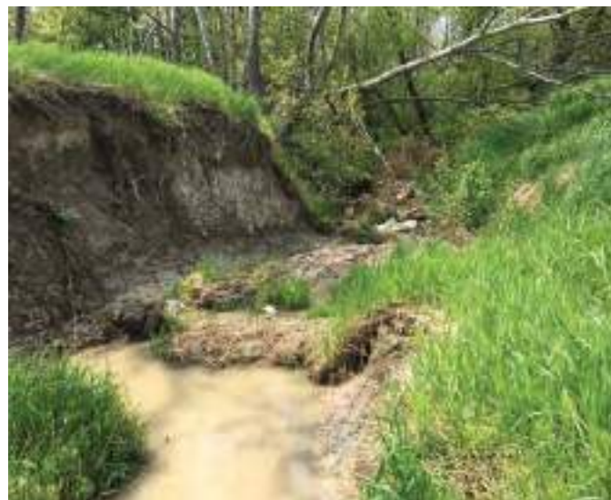
Figure B4-3. Sediment in a drain caused by failure of the drain bank.
