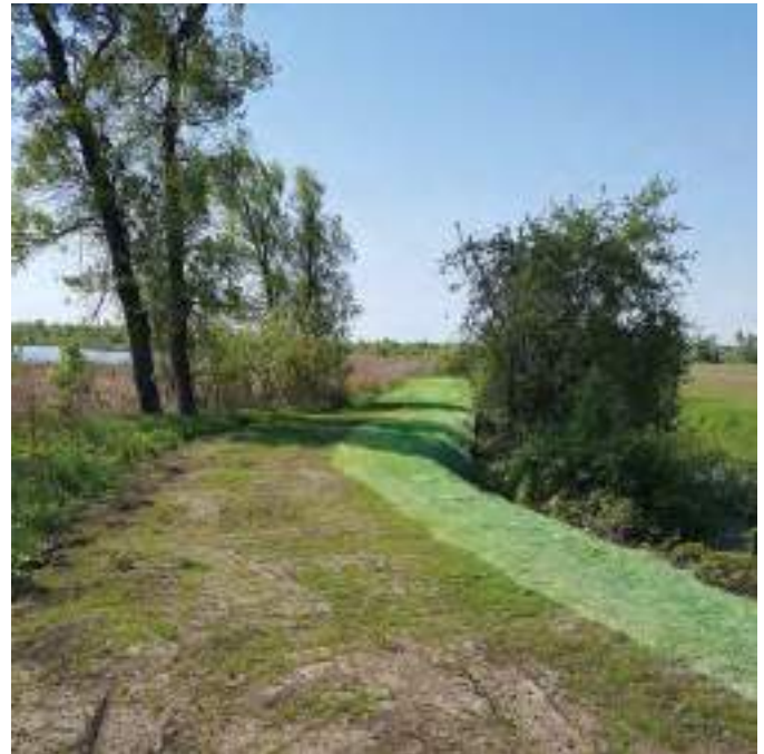
Figure A3-9. A recently repaired dyke.
