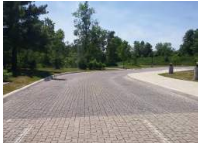
Figure B4-23. Permeable paving is used to increase the infiltration of water.
