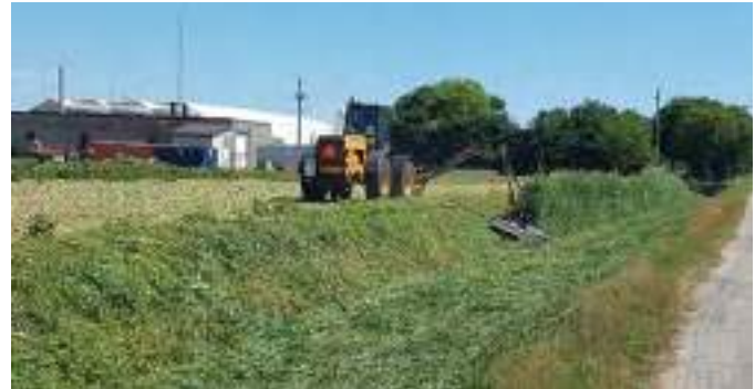
Figure B5-26. Kingsville – cutting phragmites in the drain with a boom mower apparatus.
