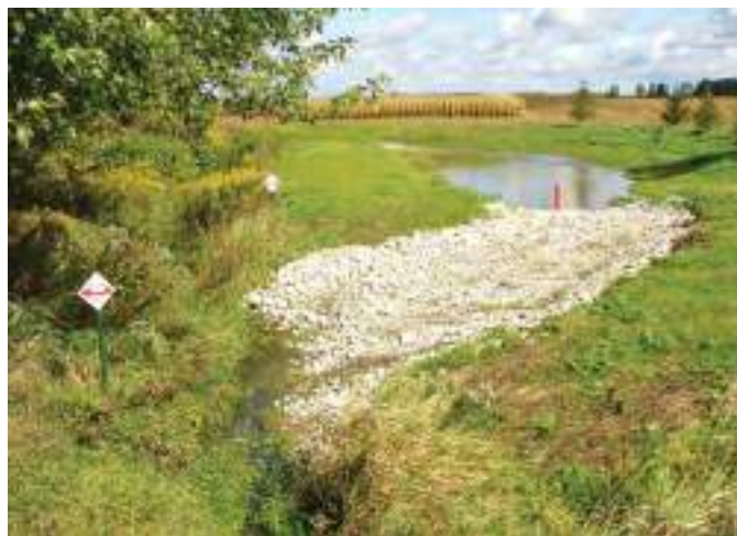
Figure B4-34. An example of an offline sediment trap. Source: Ausable Bayfield Conservation Authority, Ontario
