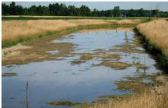
Figure B4-35. Self-forming channel (after construction). Source: Jon Witter, Ohio State University, Ohio, USA
