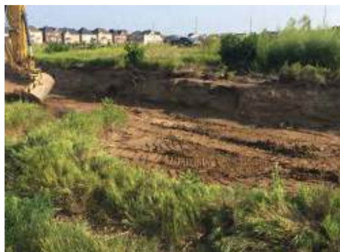
Figure B4-26. Native vegetated sod mats – donor site Source: R&M Construction, Acton, Ontario
