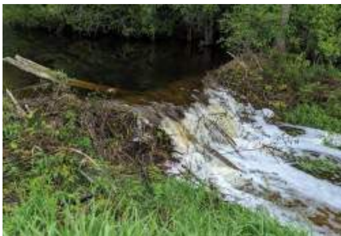
Figure A3-24. Gradual release of a dam. Source: City of Kawartha Lakes, Ontario
