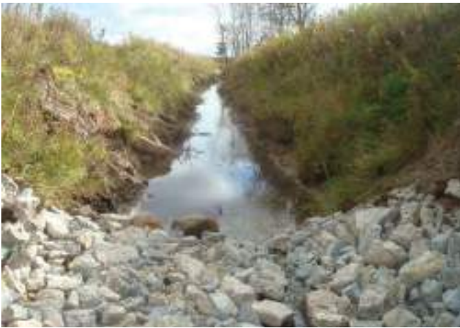
Figure B4-9. A rock check dam installed in a drain. Source: Tulloch Engineering, Espanola, Ontario
