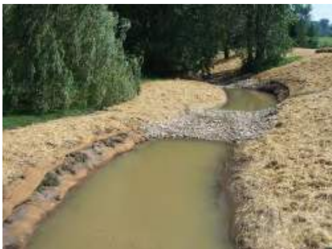
Figure B5-9. Steenstra Drain – Channel stabilization, riffle/pool sequences for fish habitat. Source: Municipality of Central Huron, Ontario
