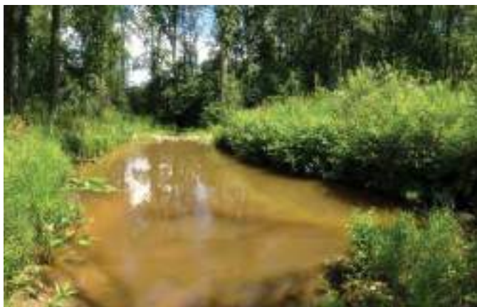
Figure B4-20. Live cribwall 2 years after construction. Source: Ian D. Smith, Lydian Environmental Consulting, Niagara Falls, Ontario
