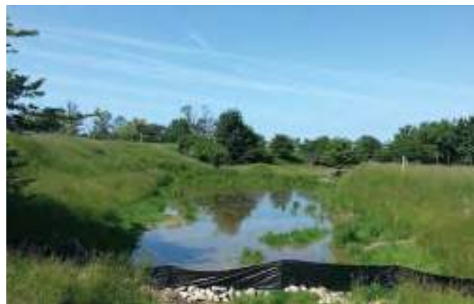
Figure B4-37. A silt fence installed next to a drain.
