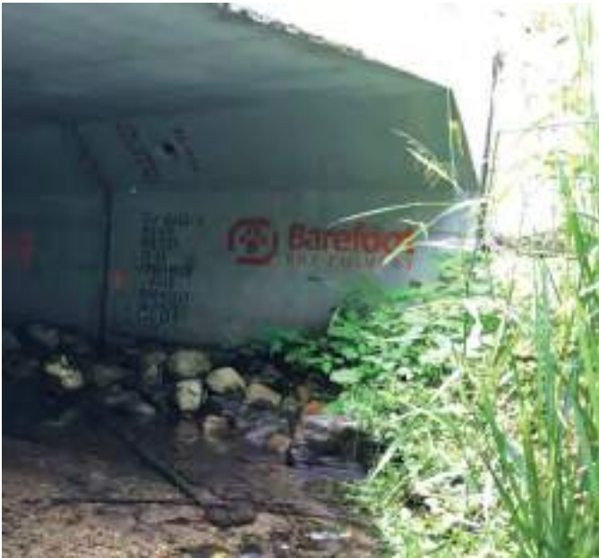
Figure B3-5. Example of green infrastructure feature – barefoot box culvert.
