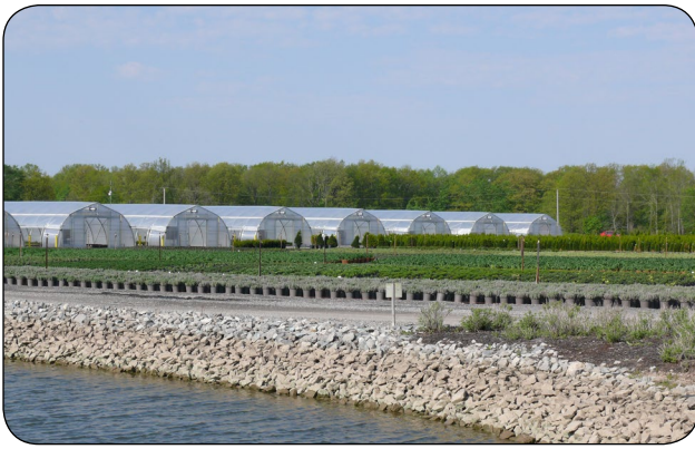
Figure 14. Rock riprap used to prevent erosion at the high water level.
