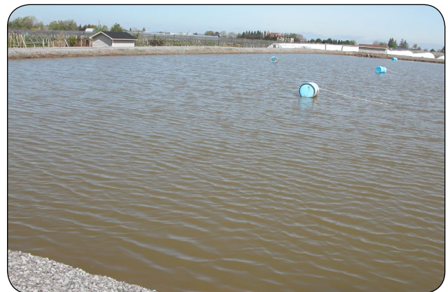
Figure 3. Example of an above grade reservoir.
