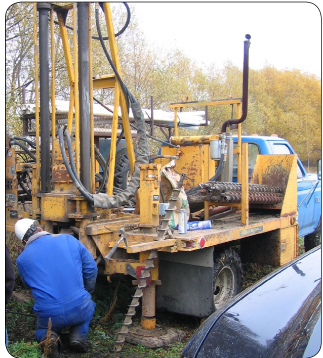
Figure 5. Drilling for clay.
