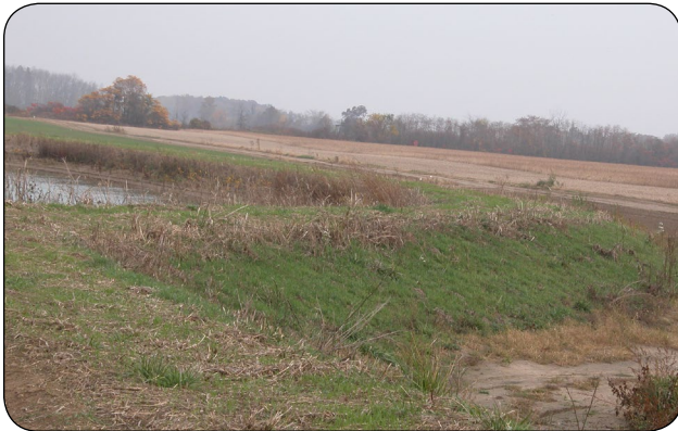
Figure 15. An above and below grade reservoir featuring a seeded bank.
