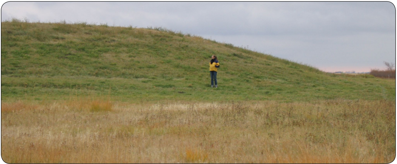
Figure 10. Example of an above and below grade reservoir.
