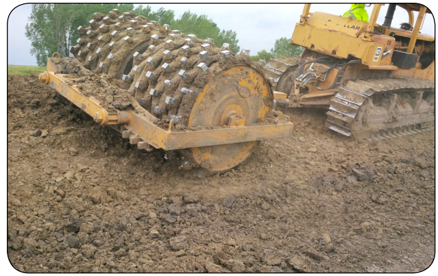
Figure 12. Compacting soil using a sheepsfoot roller.
