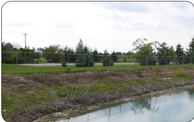
Figure 19. Safety fencing installed around the entire reservoir.
