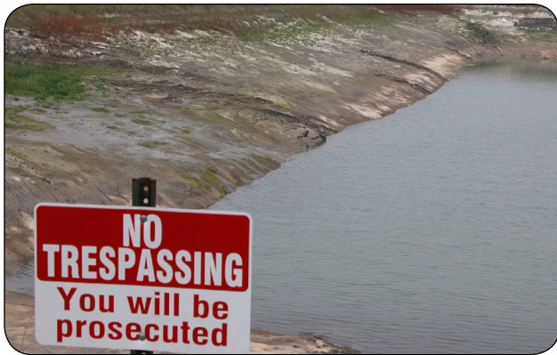
Figure 18. No trespassing sign posted at a reservoir.
