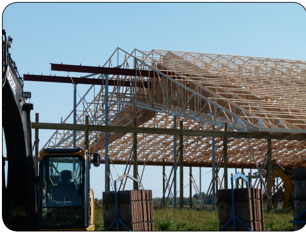
Figure 2. A barn under construction.
