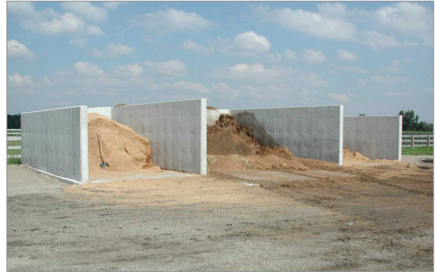
Figure 2. Example of a concrete walled structure that can be used for manure storage.
