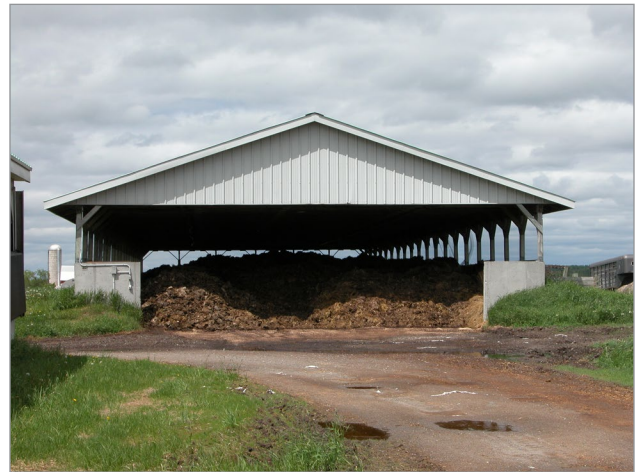
Figure 4. Covered solid nutrient storage.
