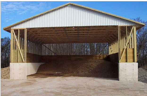
Figure 1. A covered, solid manure storage reduces or eliminates runoff.
