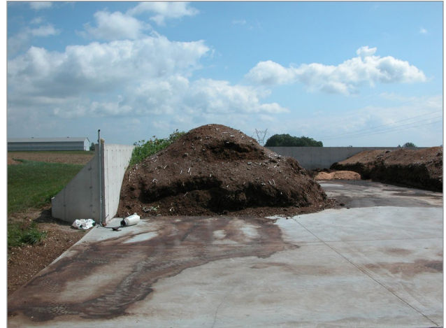
Figure 3. Runoff generated from a solid manure storage.
