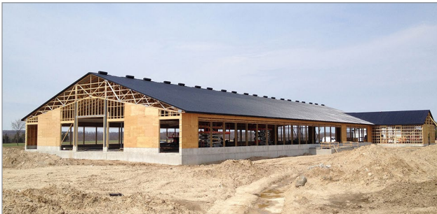
Figure 1. A building permit was required before construction started on this new livestock facility. Source: Tacoma Engineering Inc., Guelph, Ontario.
