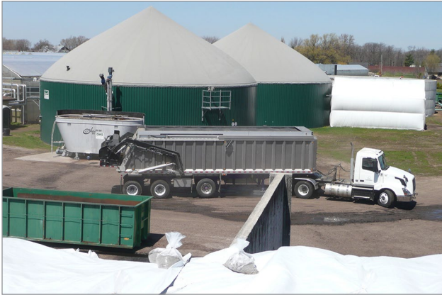
Figure 2. A load of vegetable byproducts is received at a farm-based anaerobic digestion system.
