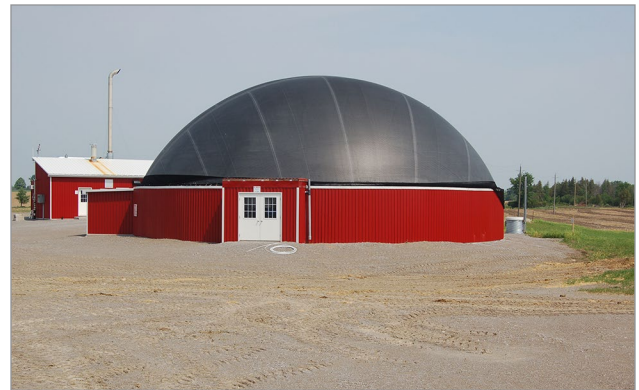
Figure 1. A manure-based anaerobic digestion system on a dairy farm.
