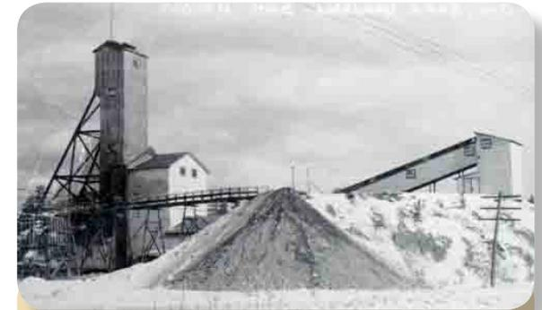
**Stop 1:** Historic photograph of the Toburn Mine during the 1940s. Waste rock from the mine was stockpiled in front of the mine. Those piles have been since quarried for construction of local roads.
