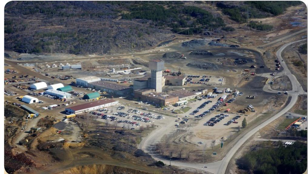
**View 7:** Aerial view of Copper Cliff (North) Mine. The concrete tower is the mine headframe. *Photo courtesy of the Ontario Geological Survey.*
