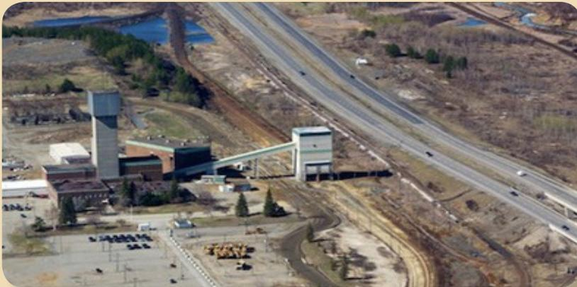
**View 2:** An aerial view of the inactive Copper Cliff (South) Mine, showing the headframe on the left. Regional Road 55 is in the upper right. When the headframe was active, ore was raised from the mine and moved by an inclined conveyor to ore bins in the white building above railway tracks, where it was loaded in rail cars for shipment to the nearby mill.
