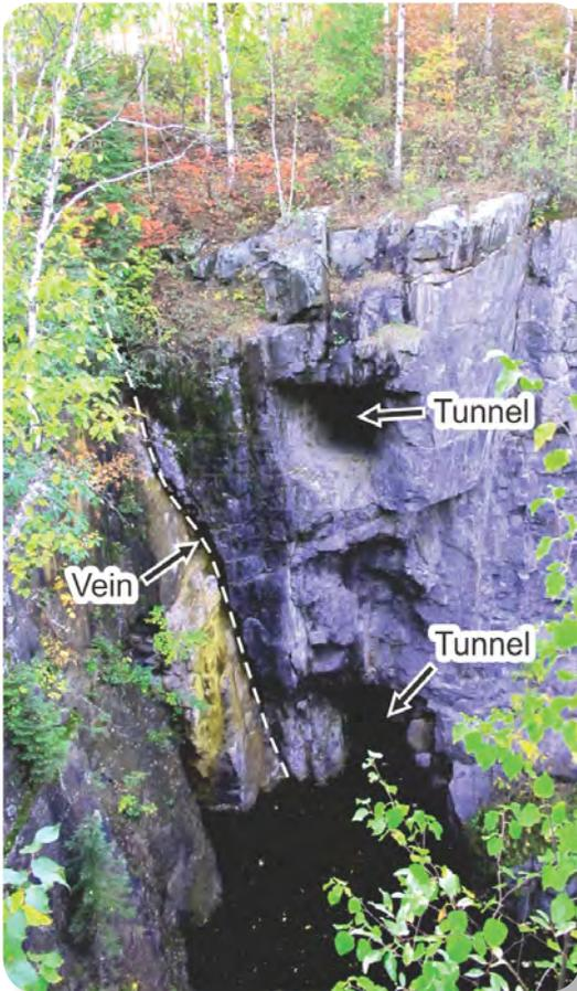
**Stop 3:** A glory hole is formed when underground mining comes to surface, creating a surface opening. This glory hole was created by mining a vein from the lower levels of the Townsite Mine. The ore was removed from below and carried in rail cars through a tunnel to the Townsite Mine shaft for hoisting to the surface. The walls of the glory hole provide a glimpse of the mine workings.
