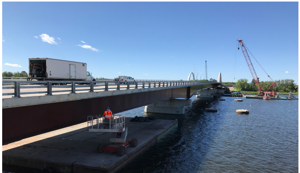
The contractor completed much of the work using large barges.
