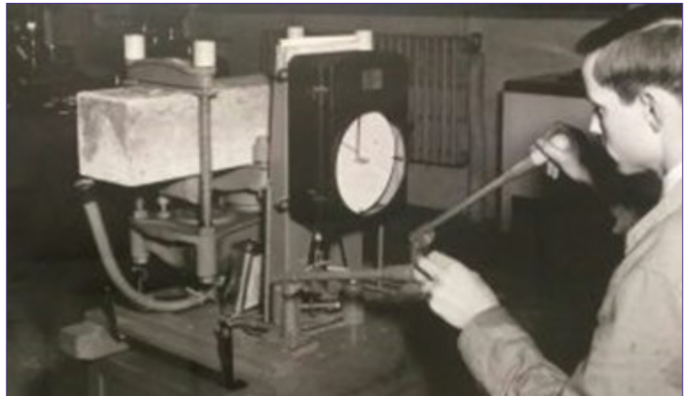
One of the many historic ministry photos displayed in the new CETI complex. This photo features a 1950's laboratory technician conducting concrete testing.
