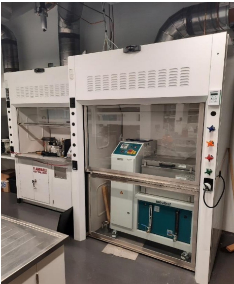
Walk-in fume Hood protects the user from fumes and vapors generated by larger apparatus. The fume hood sash goes from floor to ceiling. Equipment is rolled inside for use.
