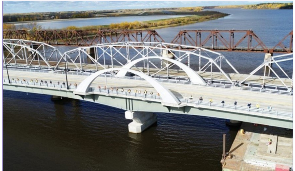
Key staff involved in the project stand six feet apart across the new international bridge.
