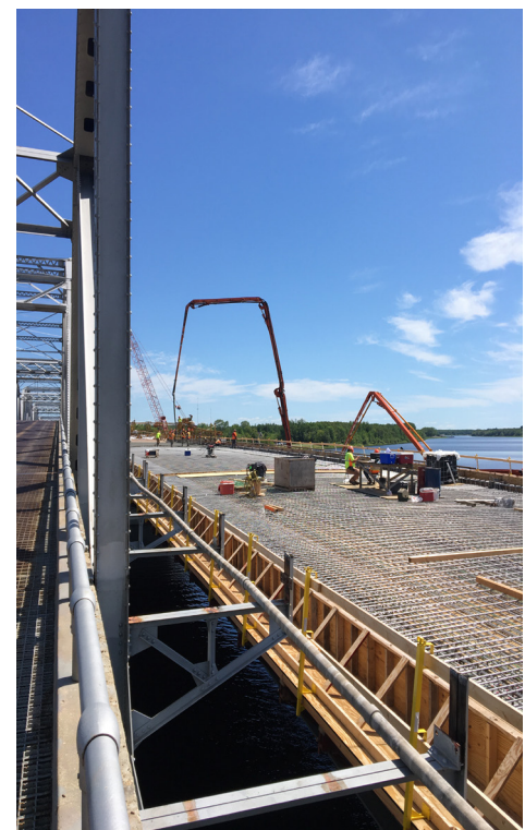
Concrete for the bridge deck is placed using concrete pumps.
