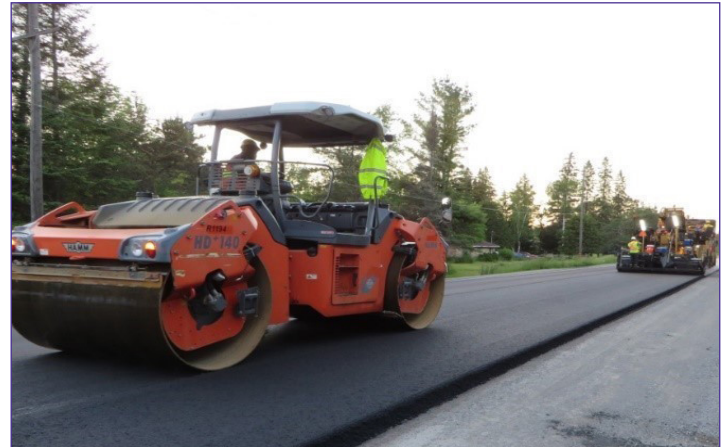
Warm Mix Asphalt paving operation showing pavement roller.
