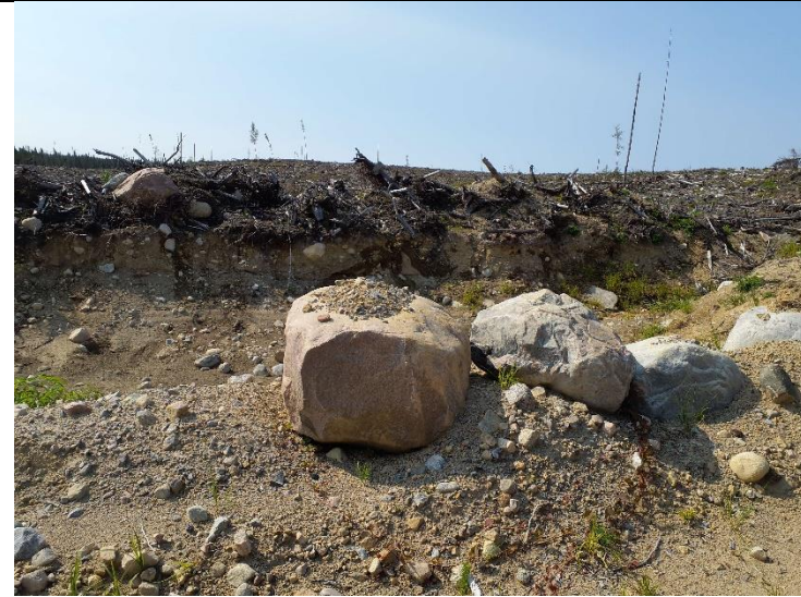
Figure 10. Inactive forestry aggregate pit adjacent an operational road. Large boulders rim the roadside face and the extraction face remains unrehabilitated.
