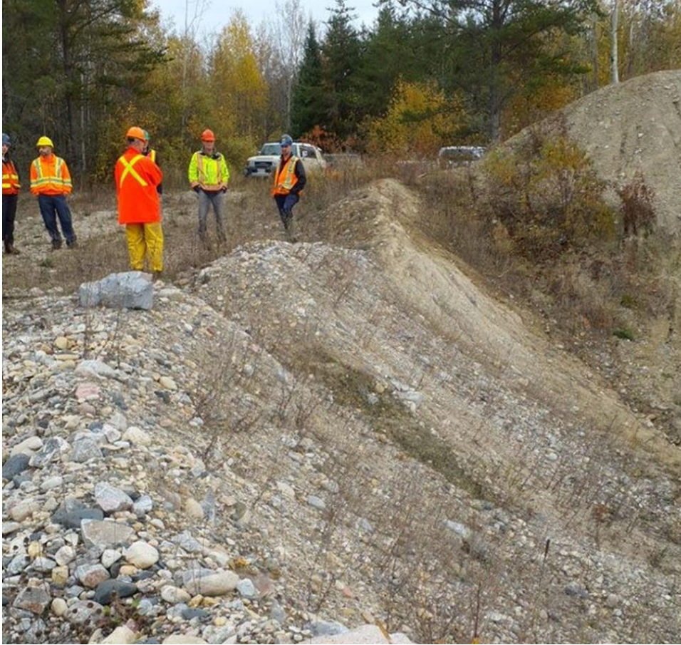
Figure 7. Runnalls Lake Area – Excavation with 15m of ditch.
