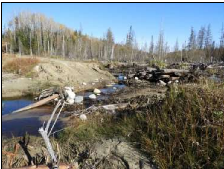
Washout on branch road of Goose Range North Rd.
