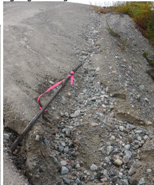
Picture #2: Road hazards and erosion caused by poor grading and extremely erodible road building material on the Stanzhinki Road.
