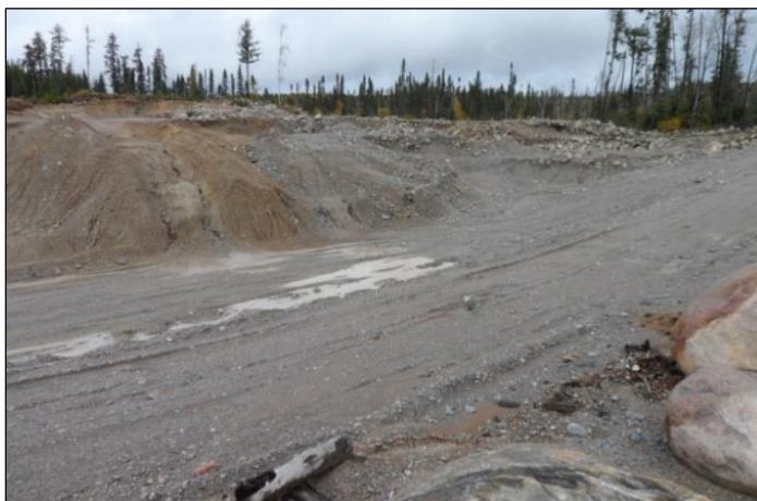
Picture #2: Pit 594L – Two unstable slopes with an overhang along the edge of the road.
