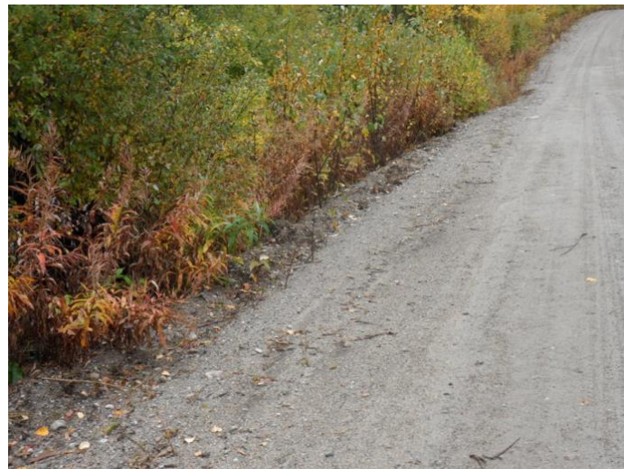
Picture #1: A false ditch has widened the road on the Race Road.
