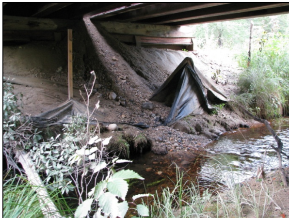
Roadbed material washing into creek under the bridge at km 17 on Ice Creek Road
