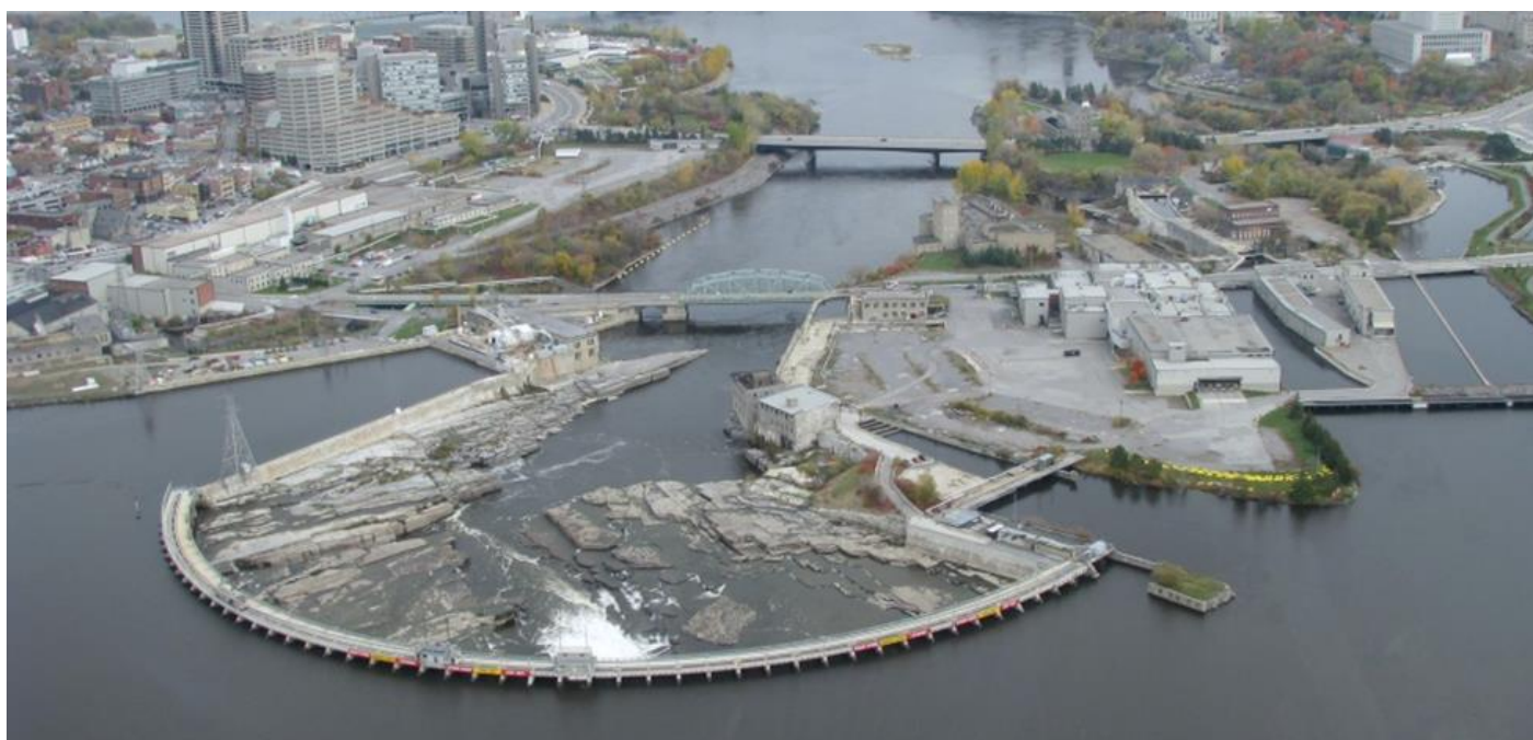
Chaudière Falls Generating Station, Hydro Ottawa, MNRF
