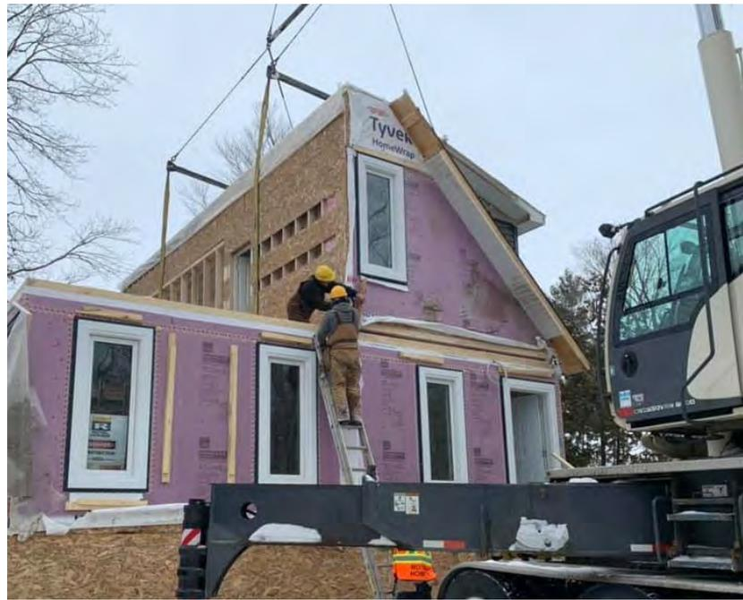
Image 9: Workers securing a second storey module into place after being moved by crane.
