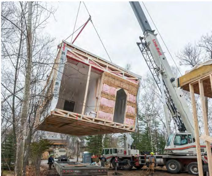
Image 13: A crane lifting a module off a flat-bed truck.
