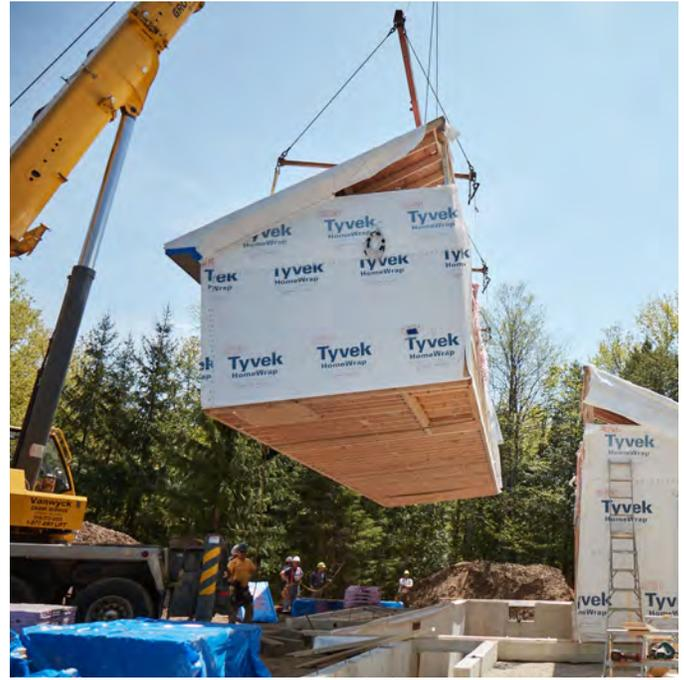
Image 1: A module being lowered by crane onto a foundation.
