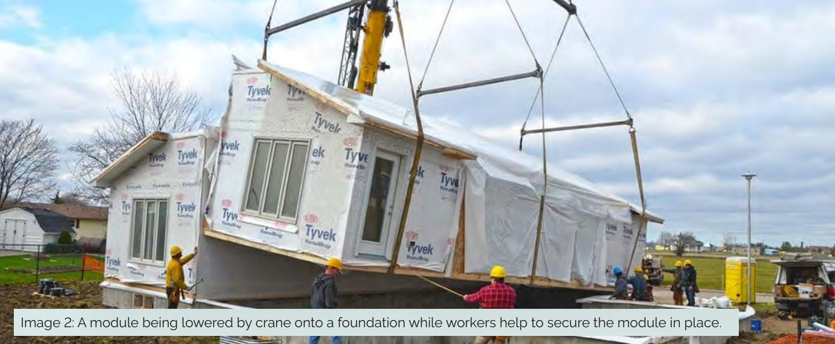
Image 2: A module being lowered by crane onto a foundation while workers help to secure the module in place.
