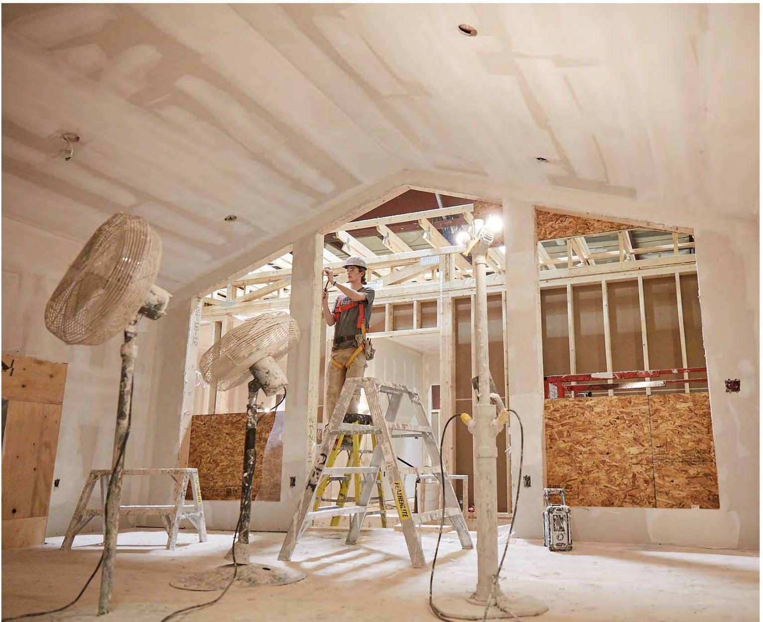
Image 16: Drywall being installed in the interior of a module.
