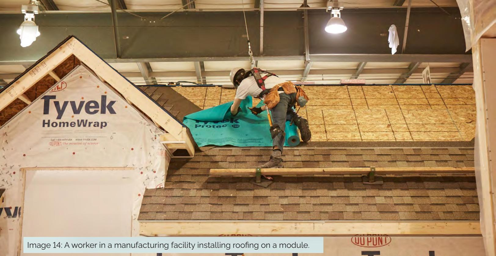
Image 14: A worker in a manufacturing facility installing roofing on a module.
