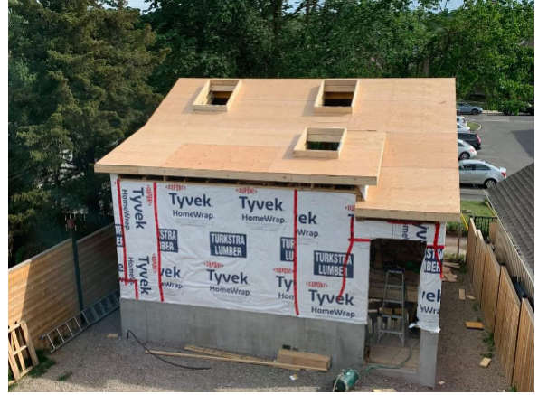
Image 6: Exterior of the laneway house
