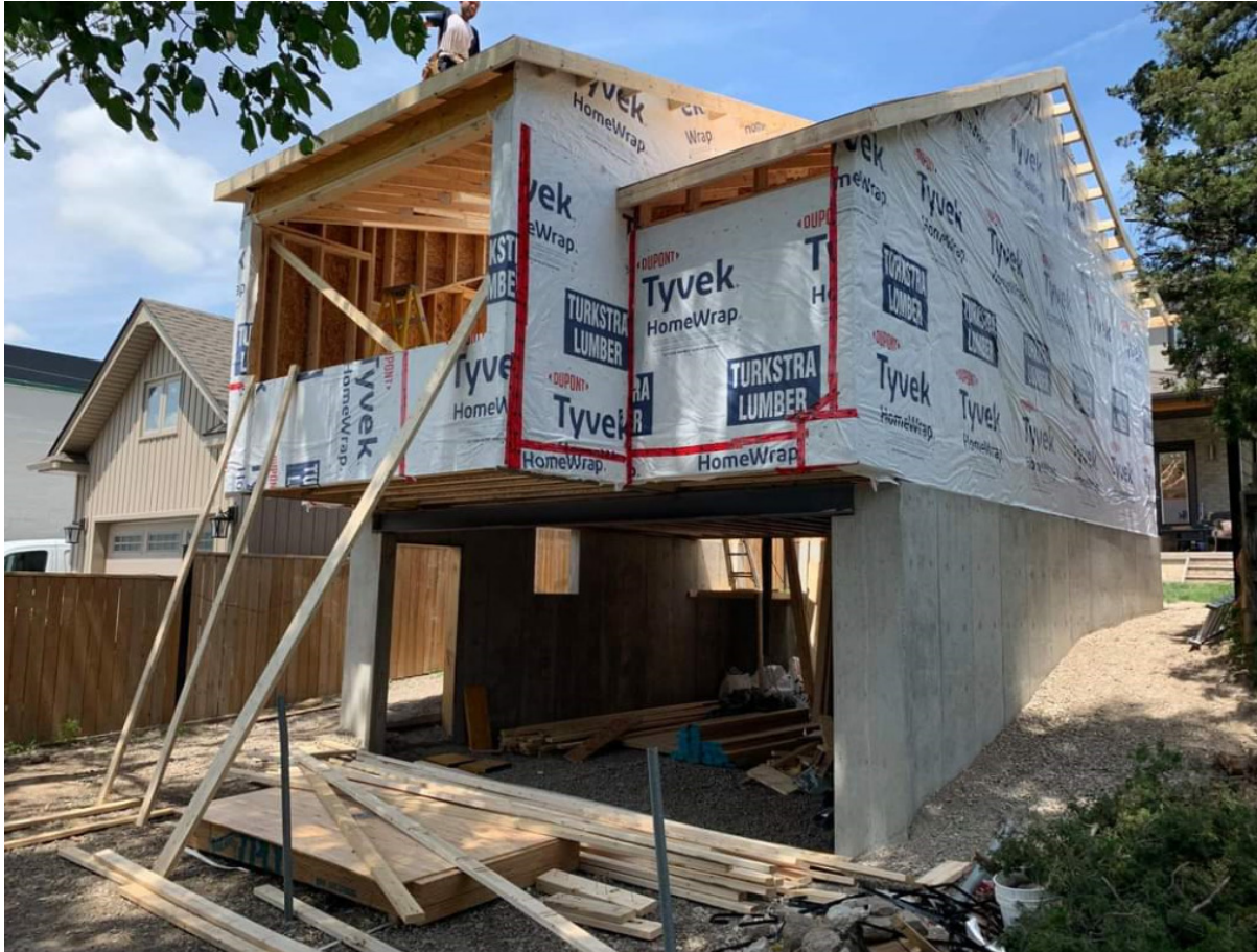
Image 7: Exterior of the laneway house
