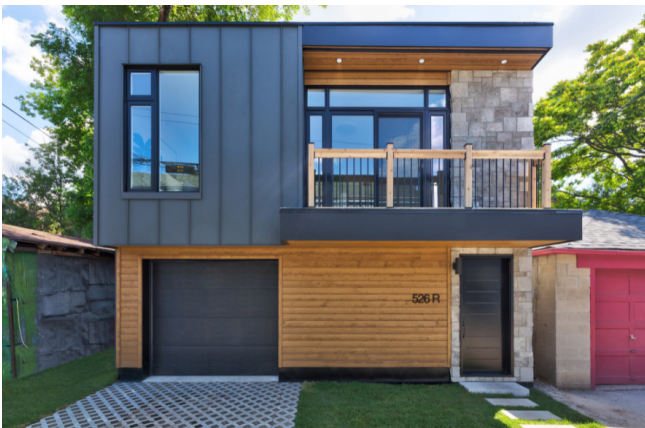
Image 5: Exterior of the laneway house
