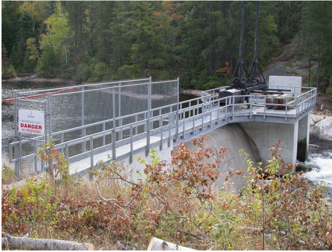
The Bannerman dam located at the south end of Onaping Lake.
