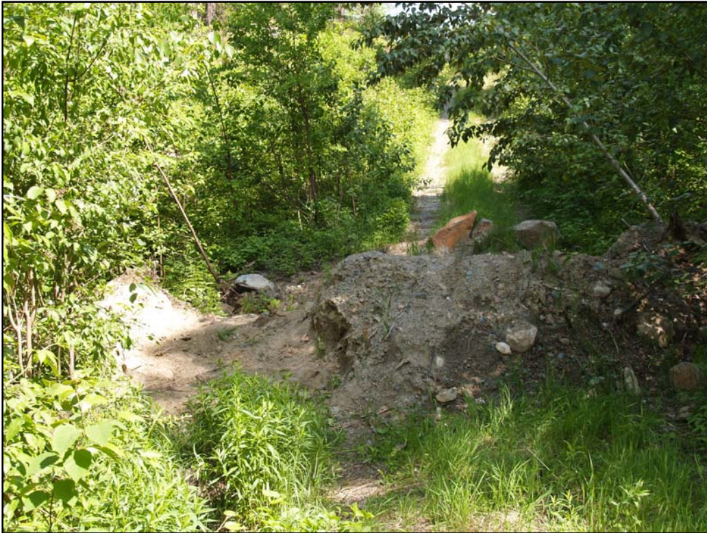
Photograph # 11. Decommissioned access road which has been breached for ATV access.
