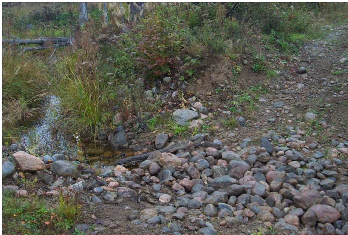
Figure 10. Decommissioned water crossing showing evidence of alteration to permit vehicle access.
