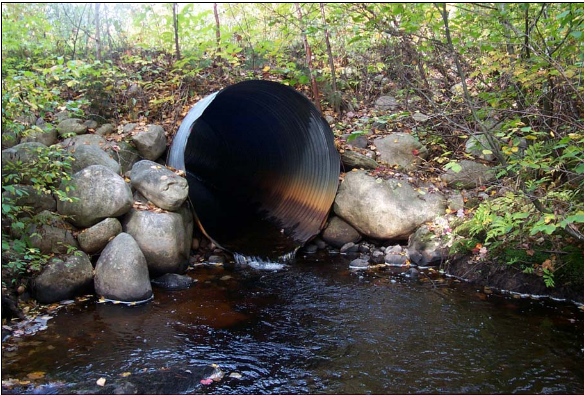
Figure 9. Perched water crossing installed prior to the audit period.
