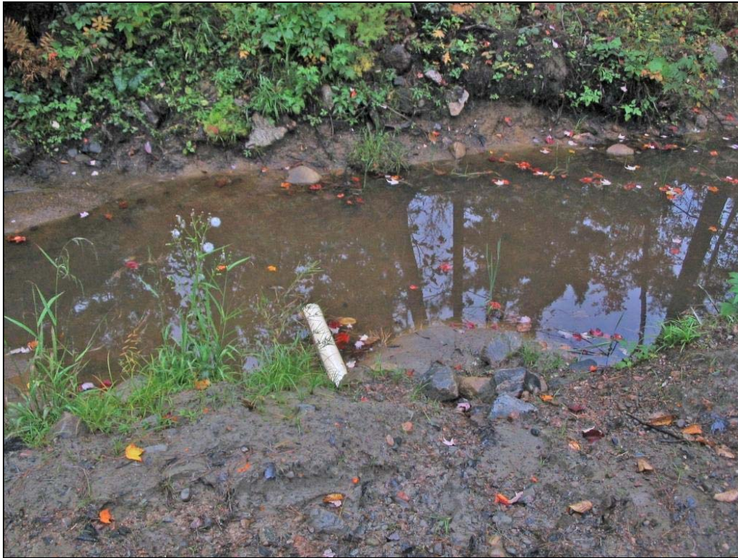
Figure 6. A four inch pipe is inadequate to allow proper drainage.
