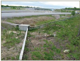
Photo 53. Fencing approaching tunnel entrance in a 'V' pattern © K. Gunson
