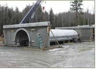
Photo 19. Arch culvert preassembled off site © K. Williams
