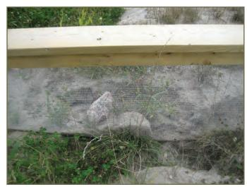
Photo 39. Hardwire cloth with ¼ inch mesh, wood frame, and top lip © K.Gunson
