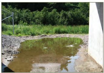
Photo 31. Water accumulation at tunnel entrance. © K. Gunson
