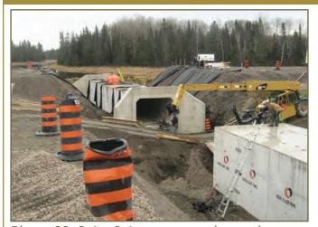
Photo 20. 3.4 x 2.4 m concrete box culvert connecting wetland habitat used by turtles on highway 69. © K. Gunson
