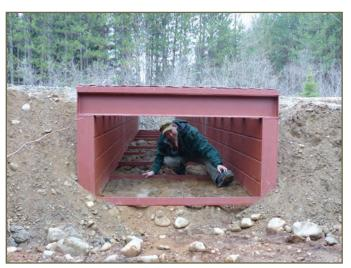
Photo 36. Tunnel structure with sediment baffles at bottom © B. Steinberg
