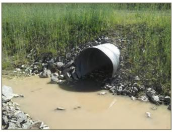
Photo 46. Pooling at culvert entrance that should be avoided at terrestrial wildlife tunnels © K. Gunson
