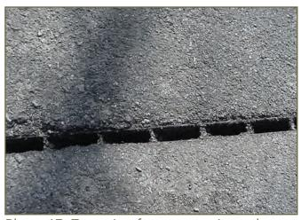
Photo 17. Zoom-in of open-top pipe culvert at road for Timber Rattlesnakes in Illinois, U.S. © S. Ballard
