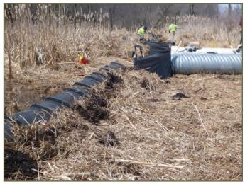
Photo 49. Backfill along ACO wildlife fence that can provide an escape ramp for animals on the roadside of the fence © V. D'elia
