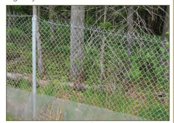
Photo 25. Small animal fence attached to the base of large animal barrier fence.
