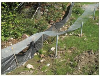
Photo 63. Temporary fencing installed prior to installation of more permanent fencing along highway 69, note permanent fencing completed in Photo 48. © W. Kowbasniuk
