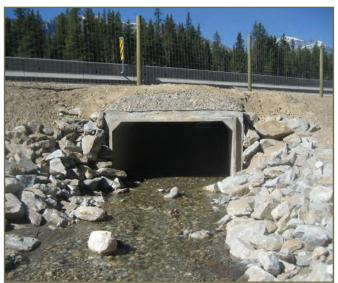
Photo 9. Open-bottom box tunnel with natural stream on Trans Canada Highway in Banff National Park, Alberta. © K. Gunson
