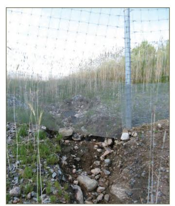
Photo 50. Fence with gap at bottom due to erosion from water draining under fence © K. Gunson
