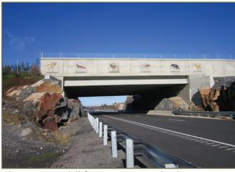
Photo 26. Wildlife overpass on highway 69 showing rock footing K. Gunson.
