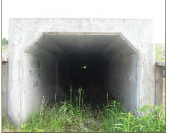
Photo 4. Open-bottom tunnel along highway 69, Ontario. © K. Gunson
