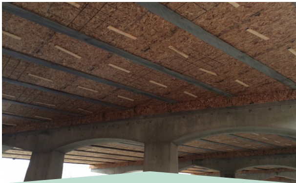
Photo 12: Underside of a bridge showing girders after installation of plywood (L. Sarris)
