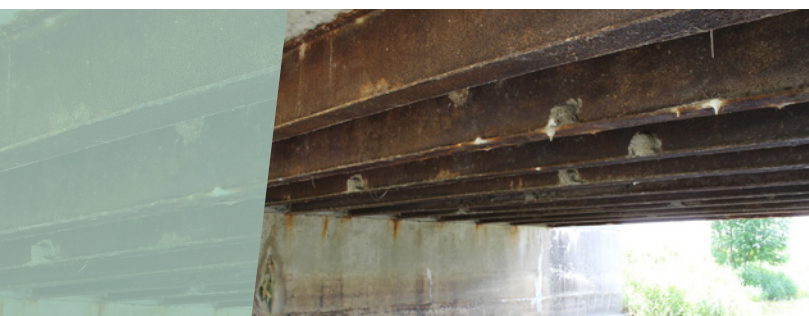
Photo 8: Barn Swallow nests on metal girders on underside of bridge over watercourse (Stantec Consulting Ltd.)
