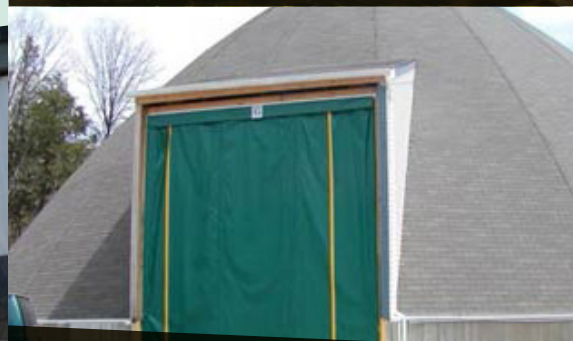
Photo 23: Curtain door on salt/sand dome storage building ( http://gatewayindustrial.com/salt-dome/doors.html )
