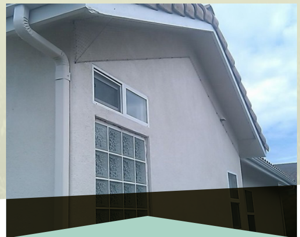
Photo 17: StealthNet® installed under the eaves of a residential building ( www.birdbarrier.com )
