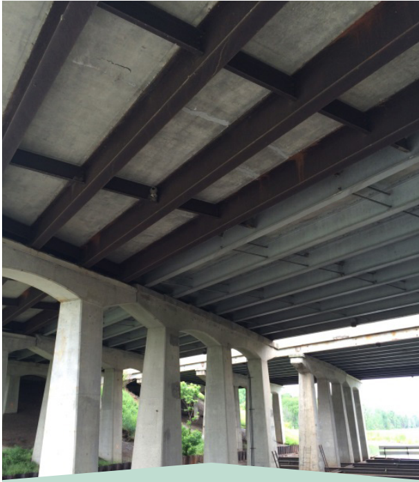
Photo 11: Underside of a bridge showing girders prior to installation of plywood (L. Sarris)
