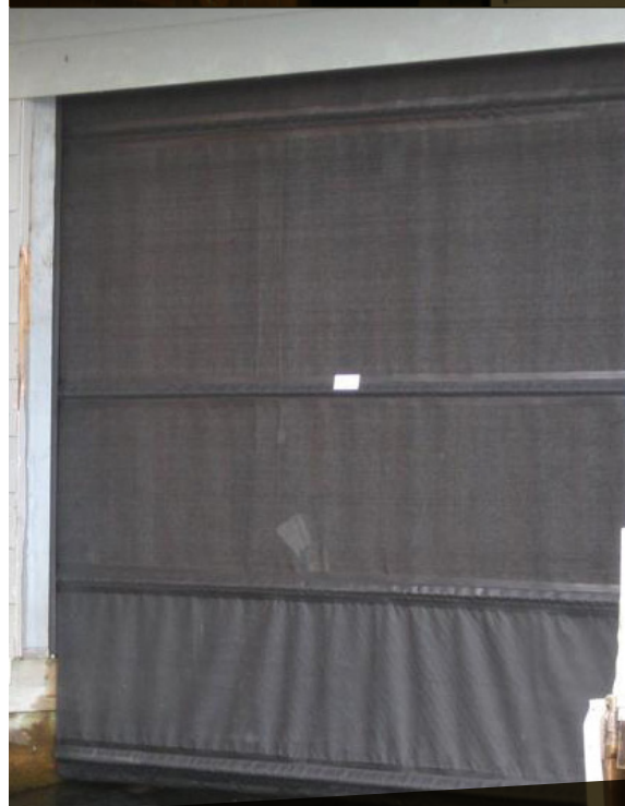
Photo 21: Curtain door installed in boathouse doorway (Marina Screen, http://www.marinascreen.com )
