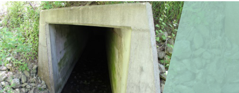
Photo 6: Entrance to concrete box culvert (Stantec Consulting Ltd.)
