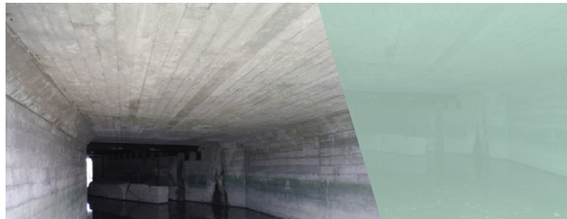
Photo 7: Large concrete box culvert (Stantec Consulting Ltd.)
