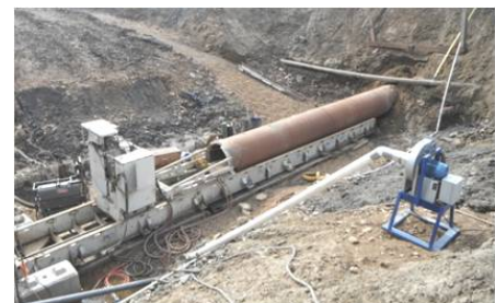
Figure 2.12: Pipe Jacking
