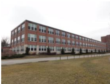
Figure 2.18: 543 Timothy Street (BHR 12) Earliest surviving component of a factory complex that extended along the tracks from Water Street to Timothy Street
