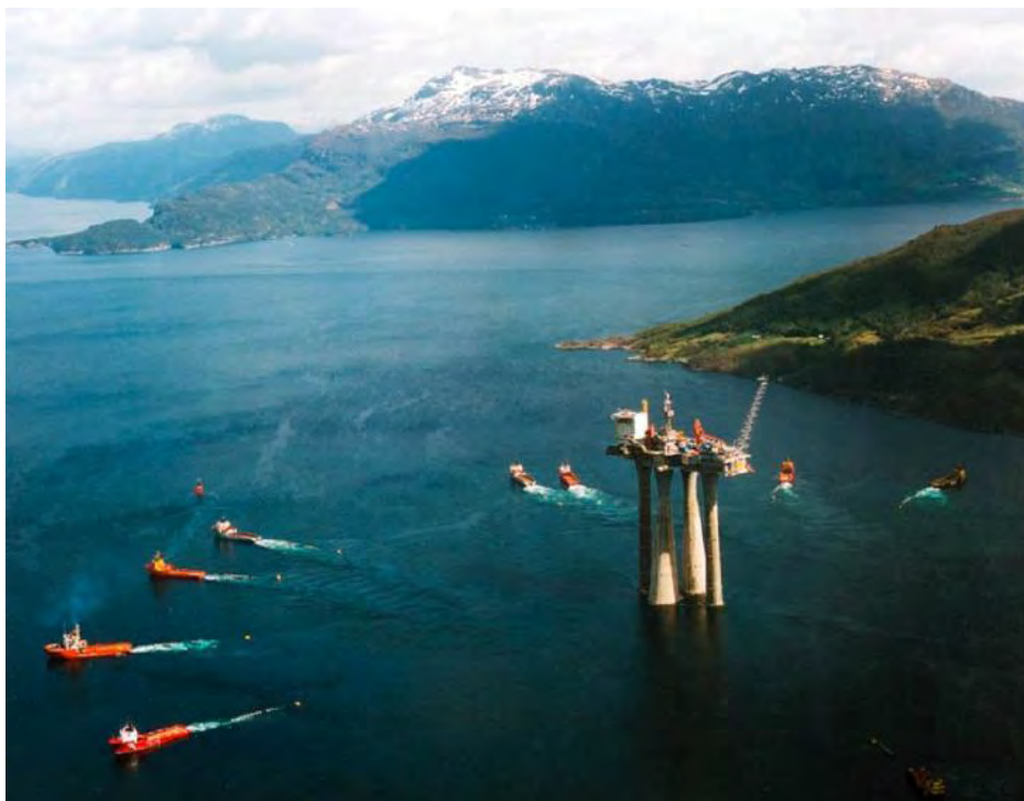
Figure 3-8 Troll A platform under tow from inshore Norway to Troll field
