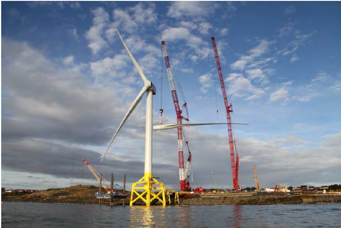
Figure 5-30 Installation of 7 MW turbine using onshore cranes
