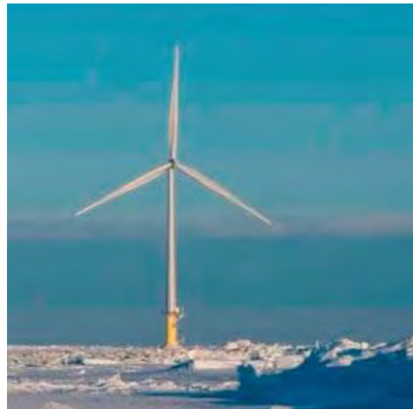
Figure 5-55 Steel GBS at Pori 1 pilot turbine
