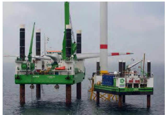
b) “Vagant” (on right) during 5 MW installation, showing relative sizes. Vagant is Seaway compliant.
