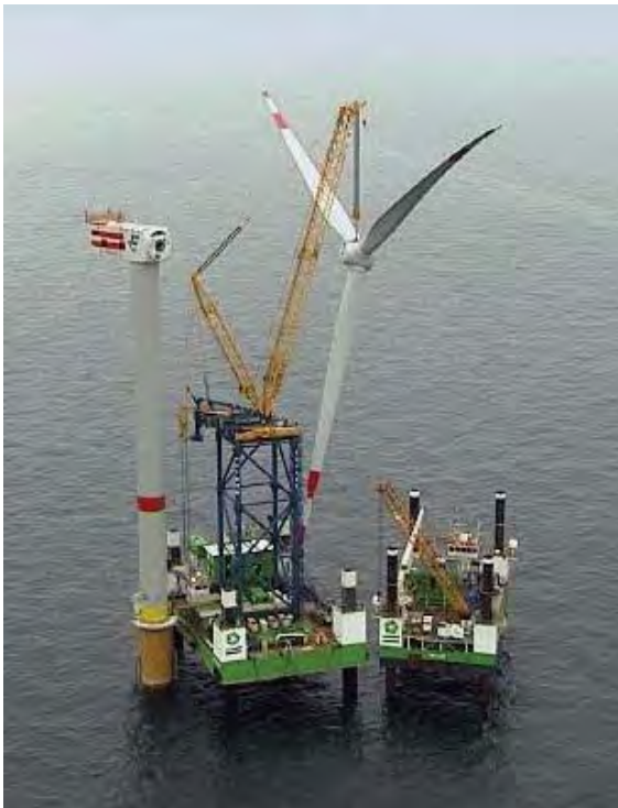
a) Custom-built gantry to raise crane on jack-up. "Buzzard" (left) and "Vagant" (right) installing 5 MW rotor star.
