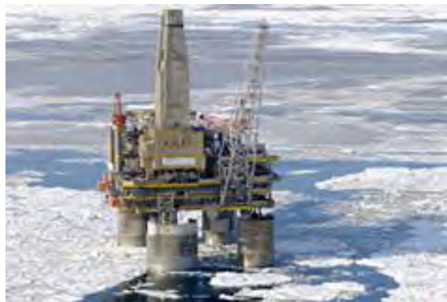
Figure 3-30 Concrete collars at Sakhalin-2 oil platform
