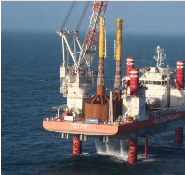
a) Met mast foundations on jack-up vessel
