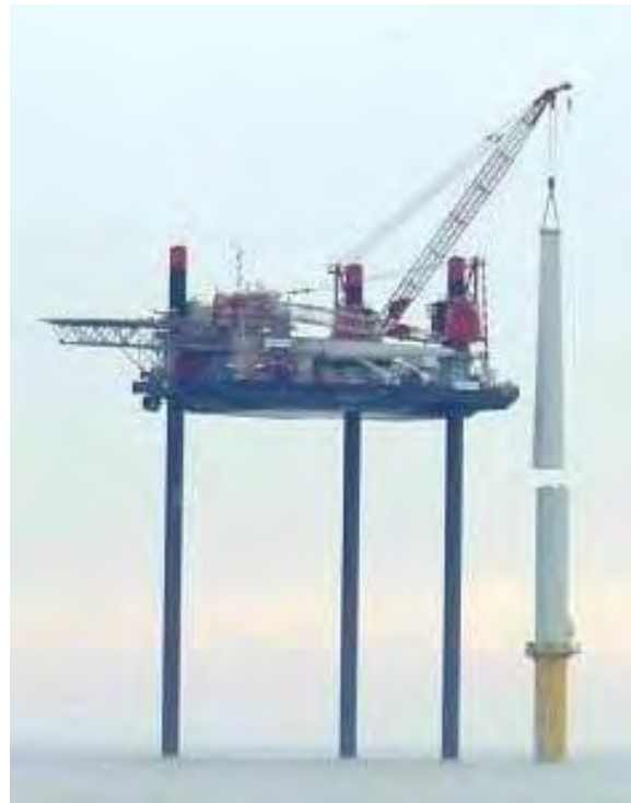
b) Use of jack-up legs in shallow water to raise crane. "KS Titan" (subsequently called "Bull Rey") installing tower.
