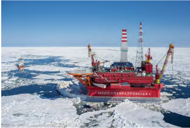
Figure 3-29 Deflector skirt at Prirazlomnaya oil platform
