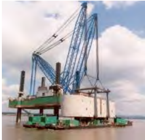
Figure 3-20 Caisson lifted by jack-up crane
