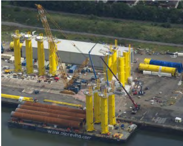
a) Loading of MPs and TPs onto barge – credit TAG
