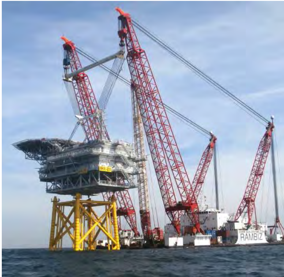
Figure 5-64 Installation of substation topside by Rambiz shearleg crane
