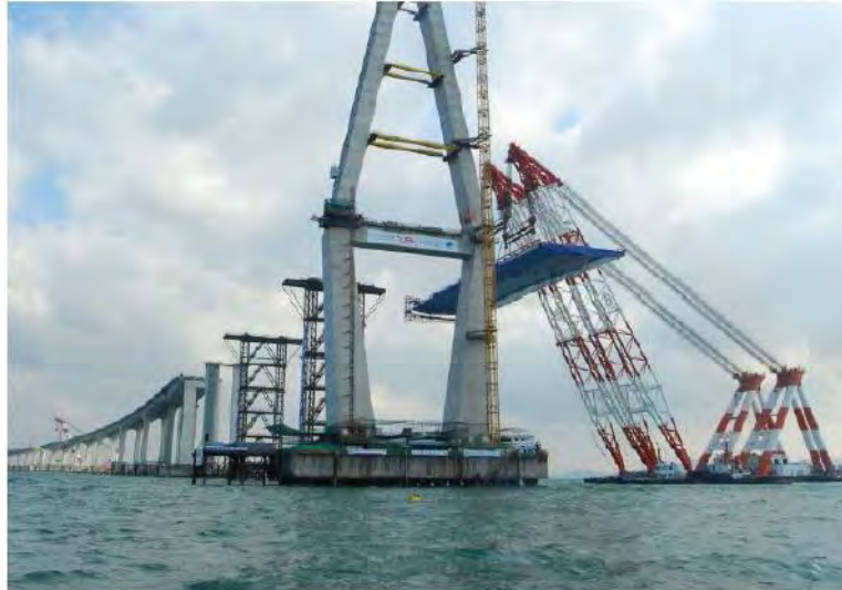
Figure 3-19 Shearleg crane vessel installing bridge span
