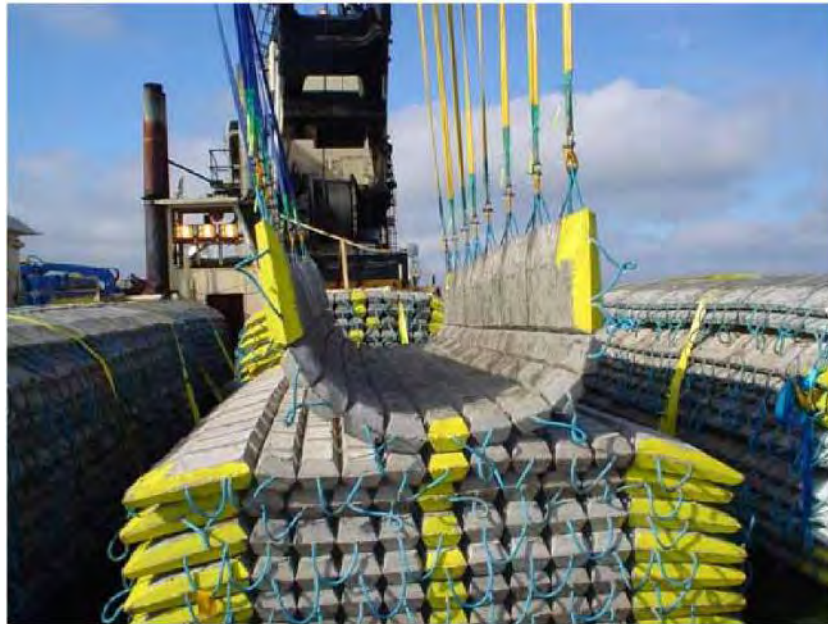
Figure 5-70 Concrete mattresses for cable protection
