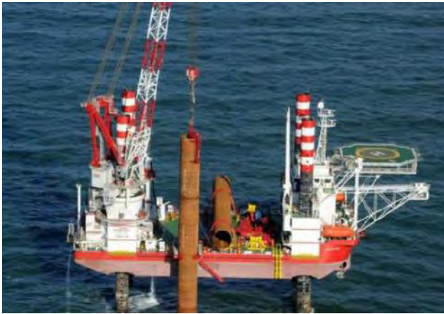
a) MP transported on crane jack-up vessel
