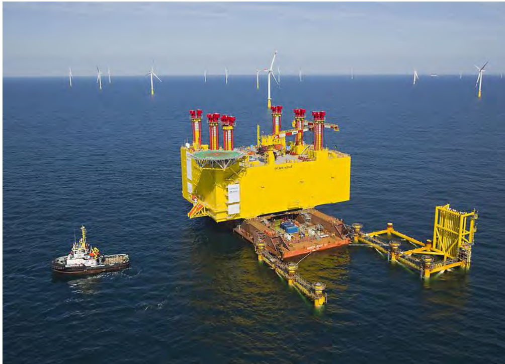
SylWin Alpha converter - credit Overdick
