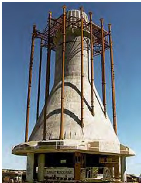
Figure 3-18 Pre-fabricated pier base for Confederation Bridge
