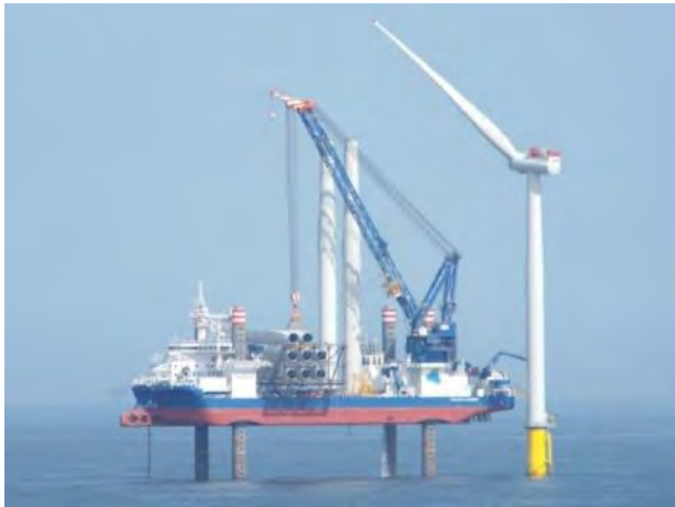
a) Jack-up vessel “Sea Challenger” installing 6 MW WTGs. 39 m beam, 132.4 m length, 900 te crane, 12 kts transit speed
