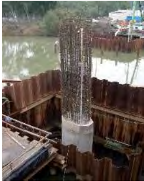
Figure 3-17 Partially cast bridge pier within caisson
