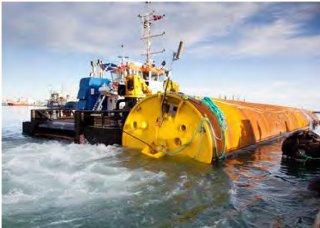
c) Towed MP showing seal – credit Dong
