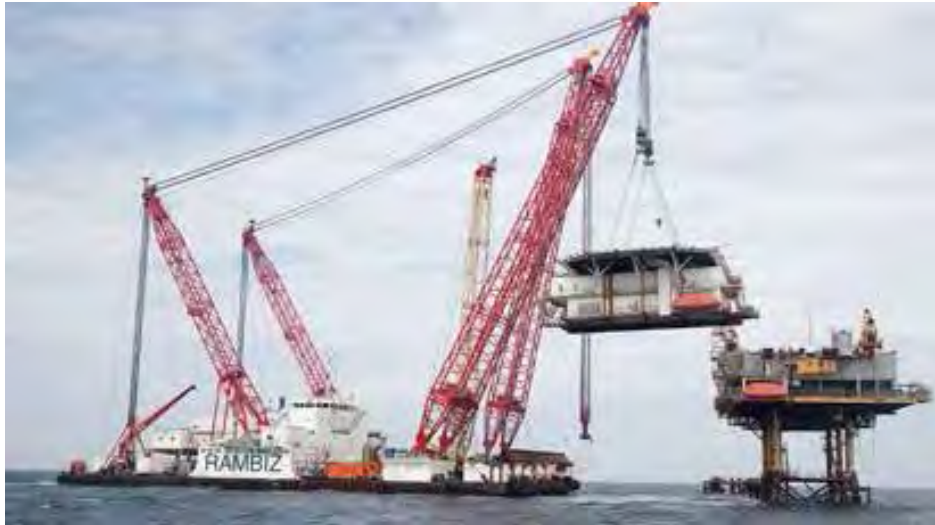
Figure 5-66 Oil & Gas sector topside decommissioning in multiple lifts
