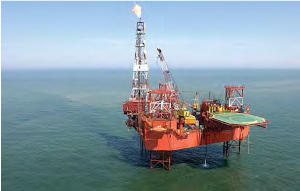
Figure 3-14 Polish oil/drilling rig in southern Baltic
