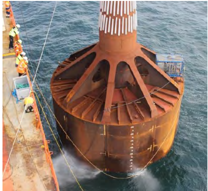
b) Installation of mono-bucket foundation
