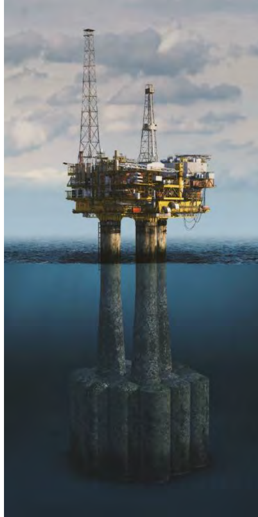
Figure 3-9 Brent gravity base O&G structure at location, showing subsea storage vessels
