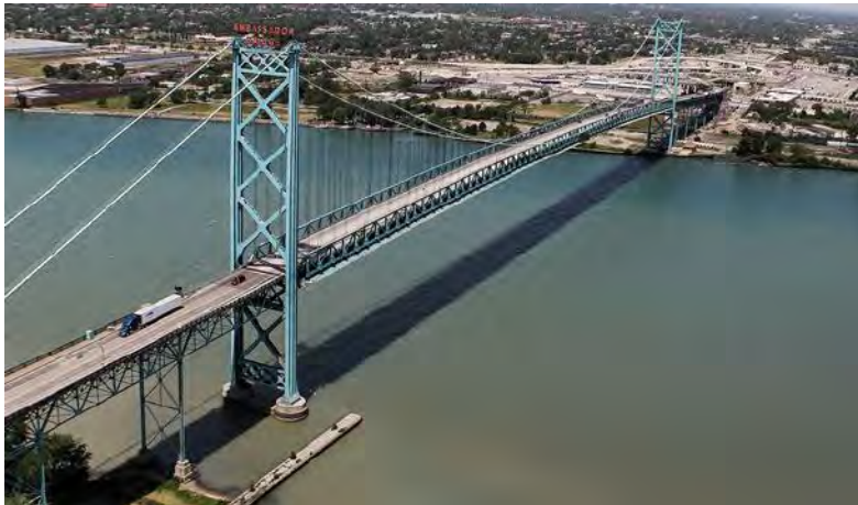
Figure 3-26 Ambassador Bridge between Detroit and Windsor, Ontario
