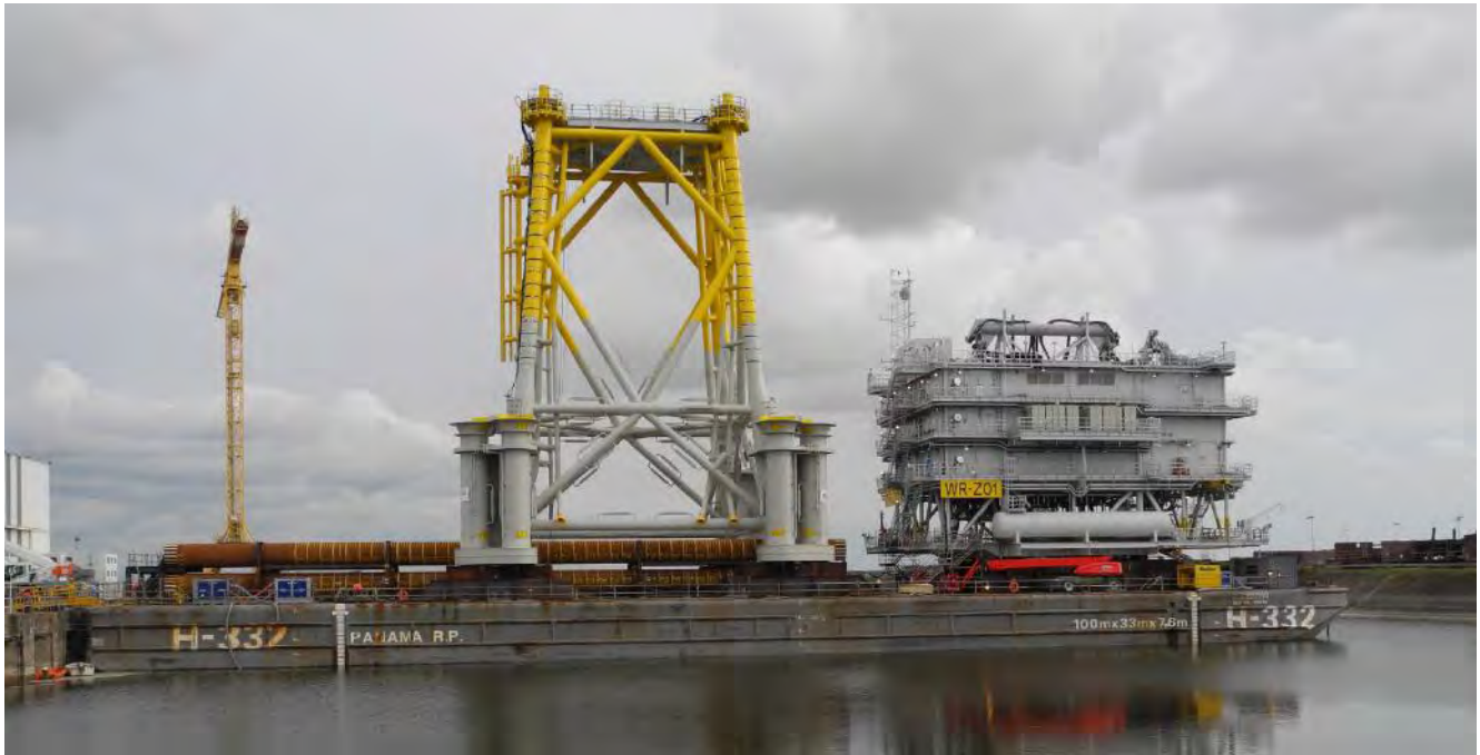
Figure 5-63 Transport of jacket and topside for offshore substation at Westermost Rough OWF
