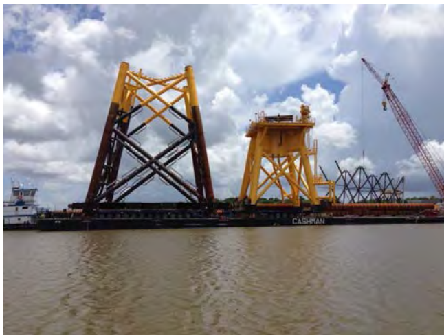
a) Two-part jacket on transport barge - credit Deepwater Wind
