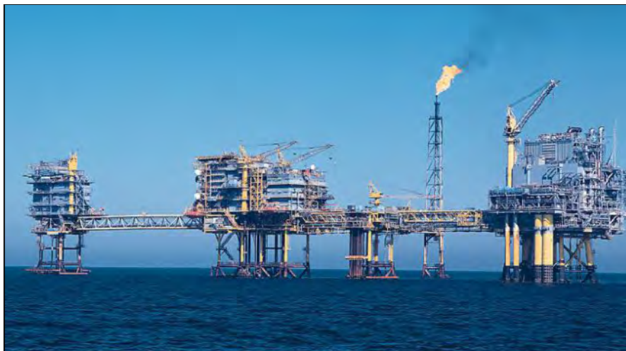
Figure 3-7 Multi-platform field complex linked by bridges
