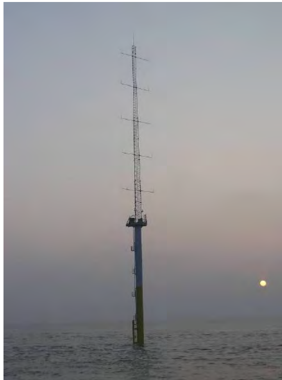
Figure 2-25 Example of offshore met mast
