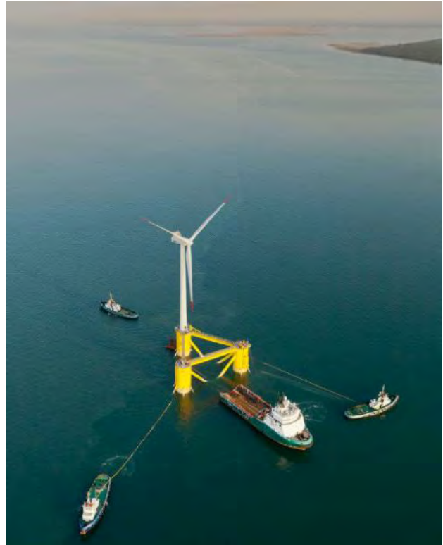
b) Tow out of complete assembly
