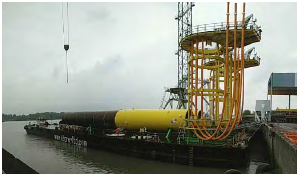
Foundations for Kentish Flats Extension - Credit Vattenfall.
