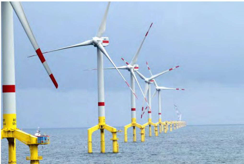
Figure 2-17 Tri-pile foundations at BARD Offshore 1
