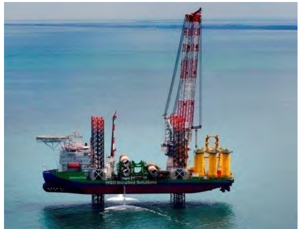
b) Jack-up vessel “Innovation” installing MPs and TPs. 42 m beam, 147.50 m length, 1500 te double boom crane, 12 kts transit speed
