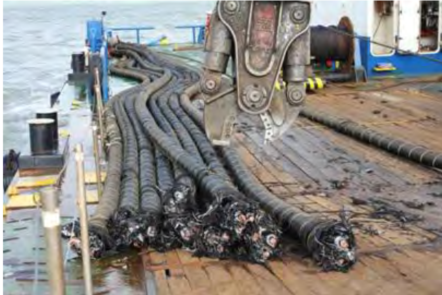
Figure 5-71 Hydraulic cutting of power cables
