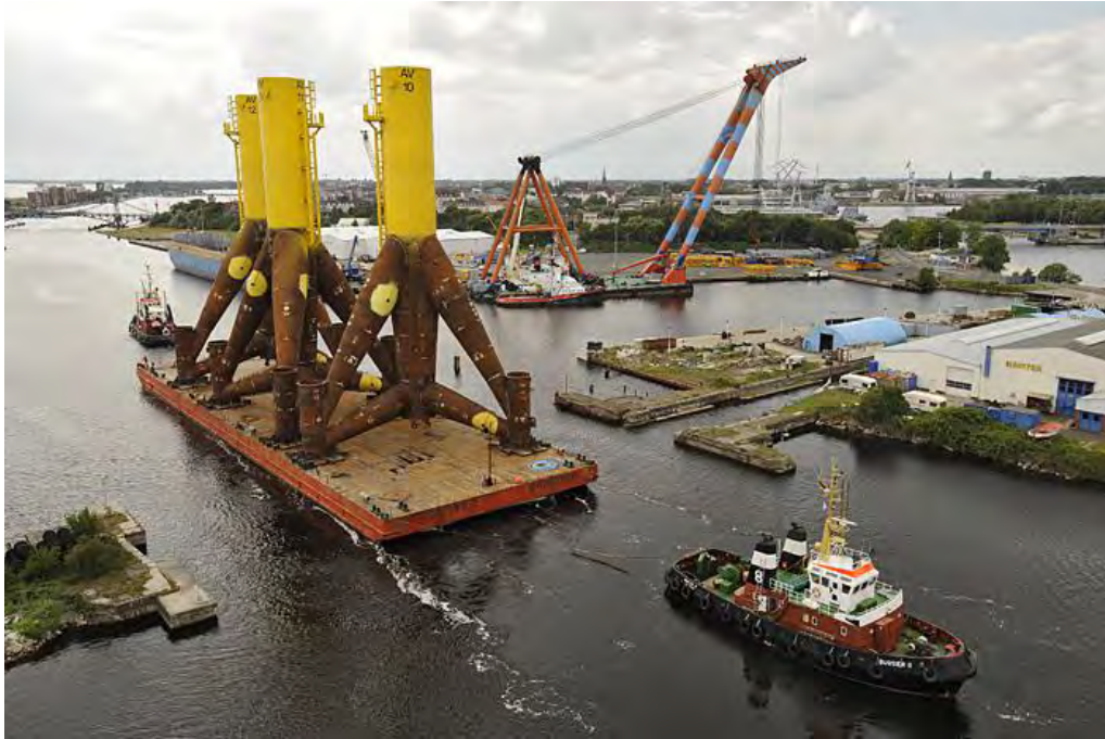
Figure 2-16 Tripod foundations for Alpha Ventus in Germany
