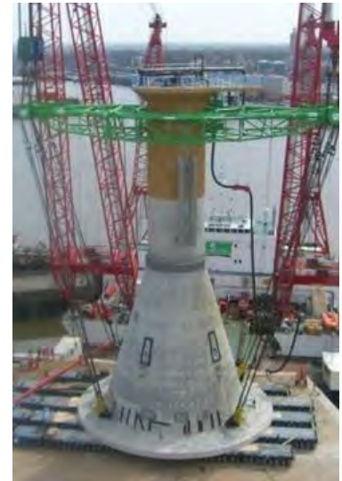
Figure 5-54 Internally ballasted GBS at Thornton Bank OWF
