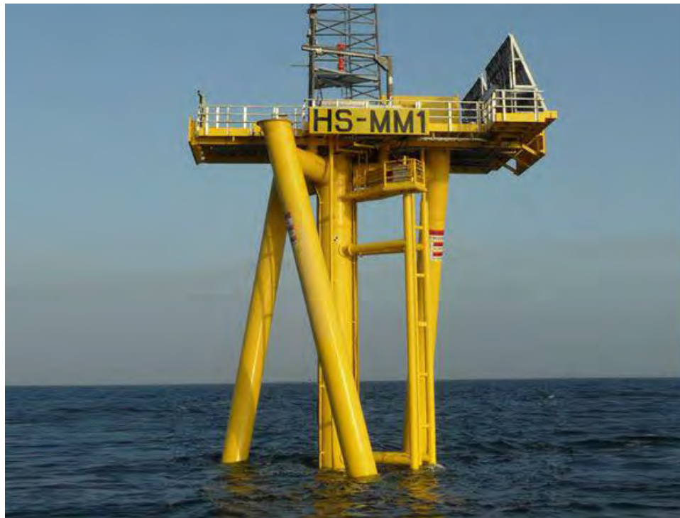
Figure 2-11 IBGS ("twisted jacket") foundation at Hornsea met mast in the UK
