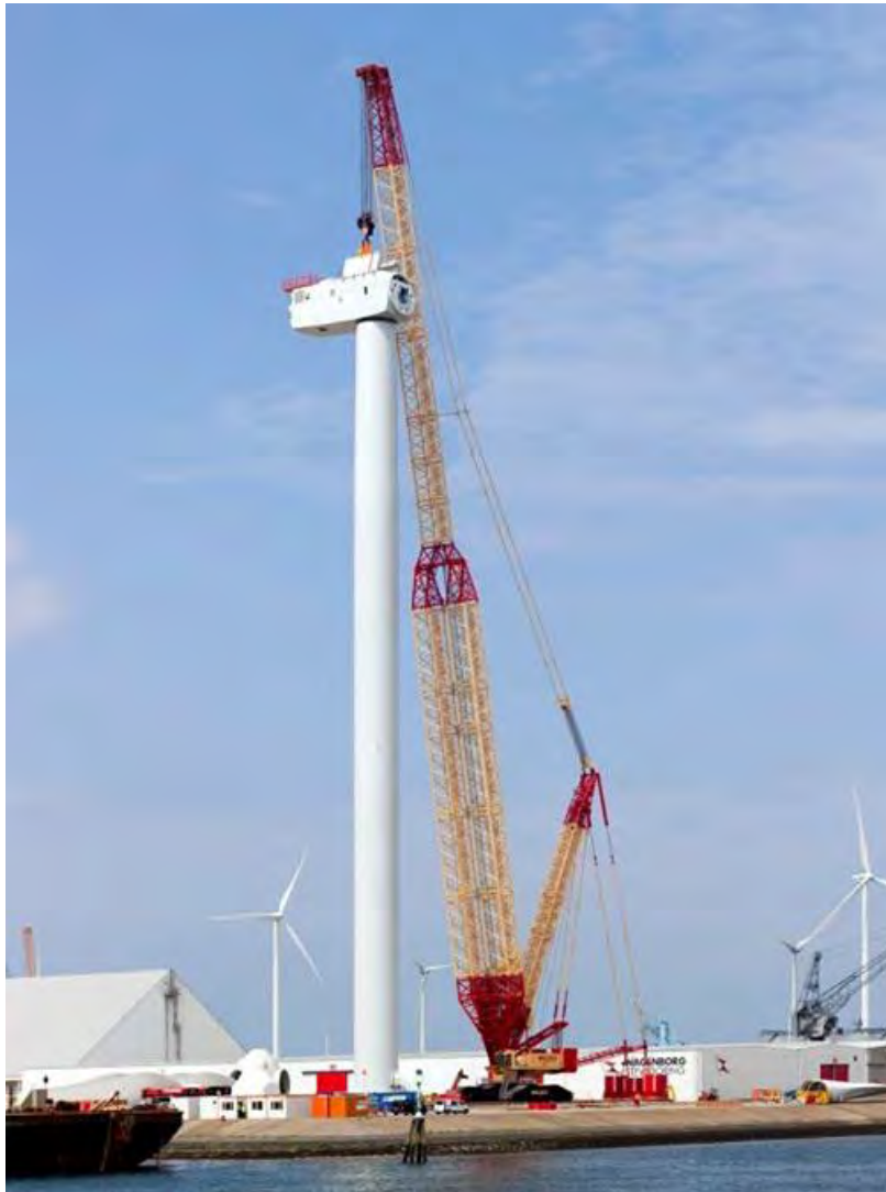
Liebherr LR 11350-P1800 lifting 340 t nacelle to 110 m – Credit Liebherr.
