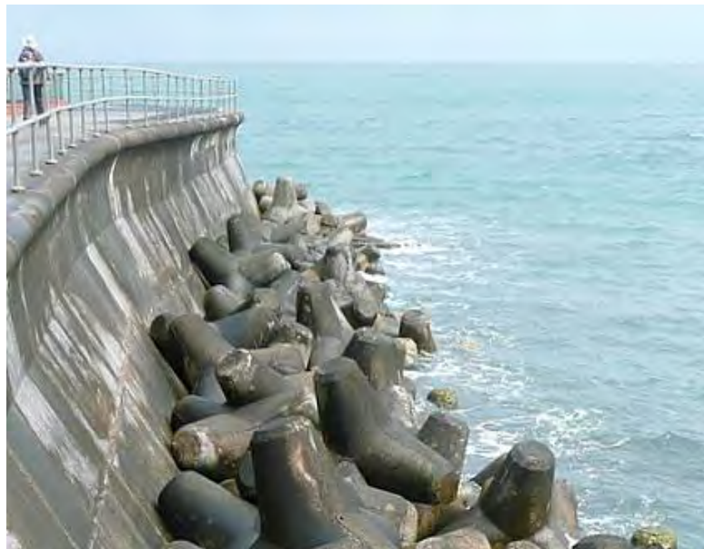
Figure 3-24 Tetrapod armour blocks providing protection from wave erosion
