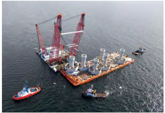
b) Installation by lift from barge at Karehamn OWF Credit - Scaldis
