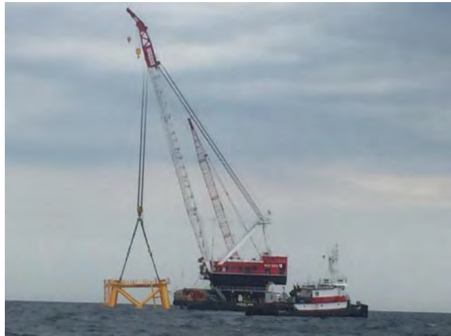
b) "Weeks 533" floating crane lifting lower jacket section into place – credit Deepwater Wind
