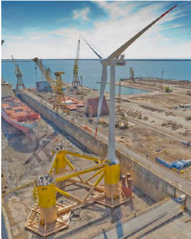
a) Assembly of platform and turbine in dry dock
