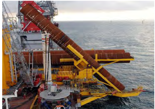
b) Upending of MP using manipulator
