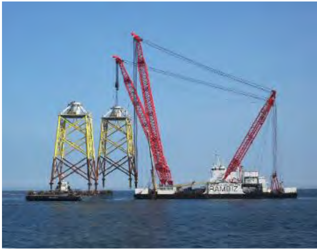
a) By floating shearleg crane – Ormonde OWF
