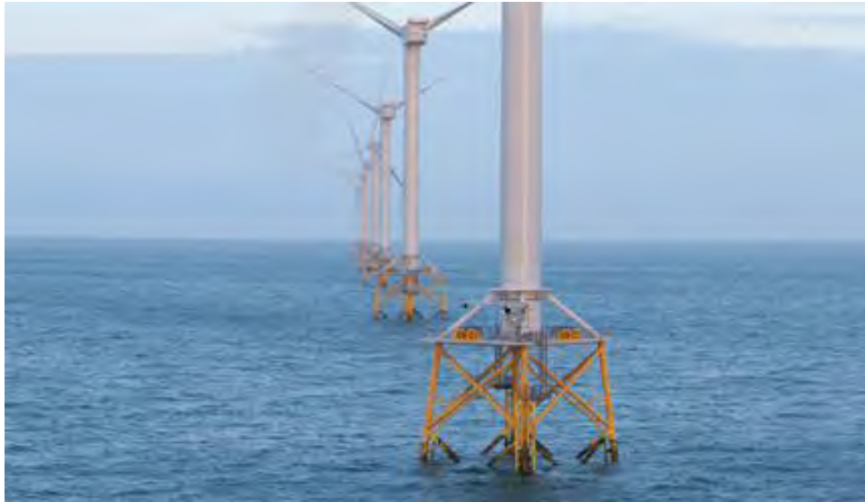
Figure 2-10 Jacket foundations at Ormonde offshore wind farm in the UK
