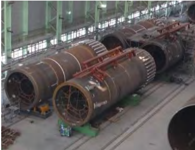
Addition of secondary steelwork to TP – credit EEW
