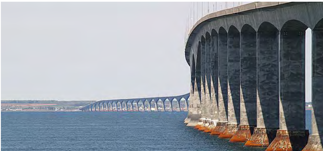
Figure 3-32 Conical ice shields at the waterline of Confederation Bridge piers
