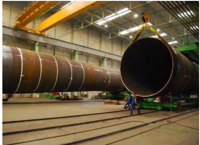
b) Welded cans forming 7.5 m diameter MP – credit EEW
