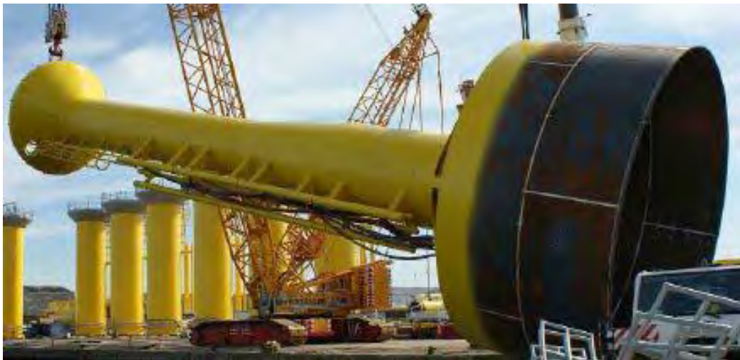
Figure 2-18 Suction bucket foundation for Horns Rev II met mast
