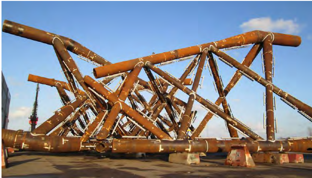
Figure 5-43 Fabrication of jacket
