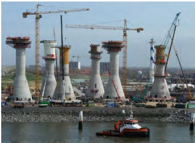
a) Construction on strengthened quayside
