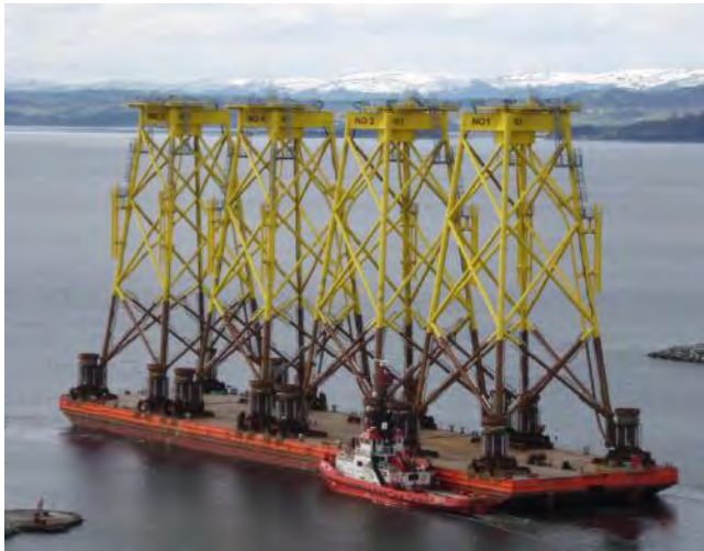
a) Nordsee Ost jackets – credit RWE
