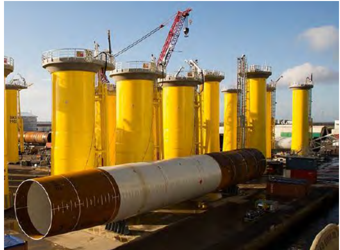
Complete MP and TPs ready for installation – credit DEME-GeoSea
