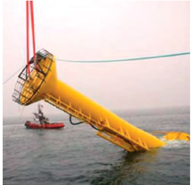
b) Upending using heave-compensated crane
