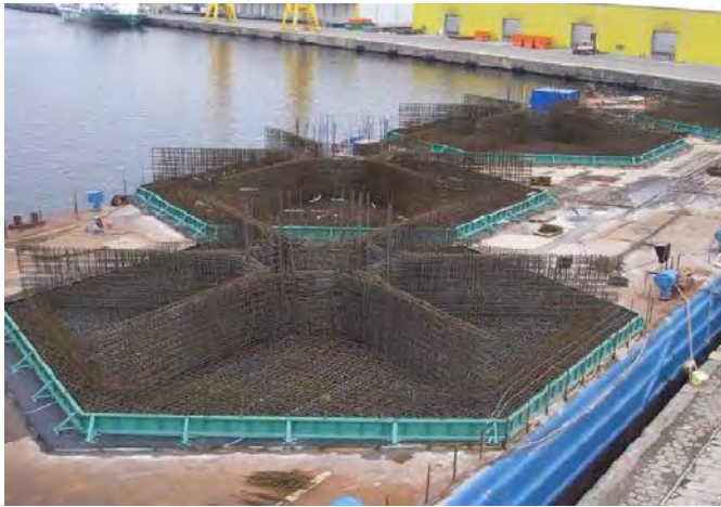
a) Reinforced concrete construction on barge, for Lillgrund OWF Credit - Hochtief
