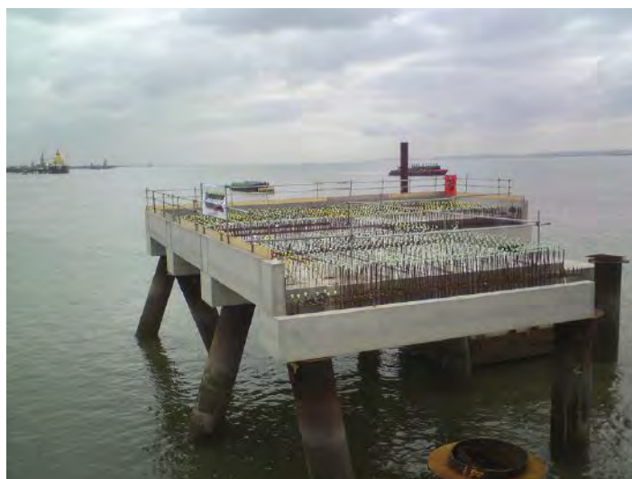
Figure 3-21 Dolphin under construction showing angled piles
