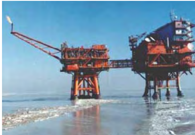
Figure 3-31 Conical ice deflectors in Bohai Bay, China
